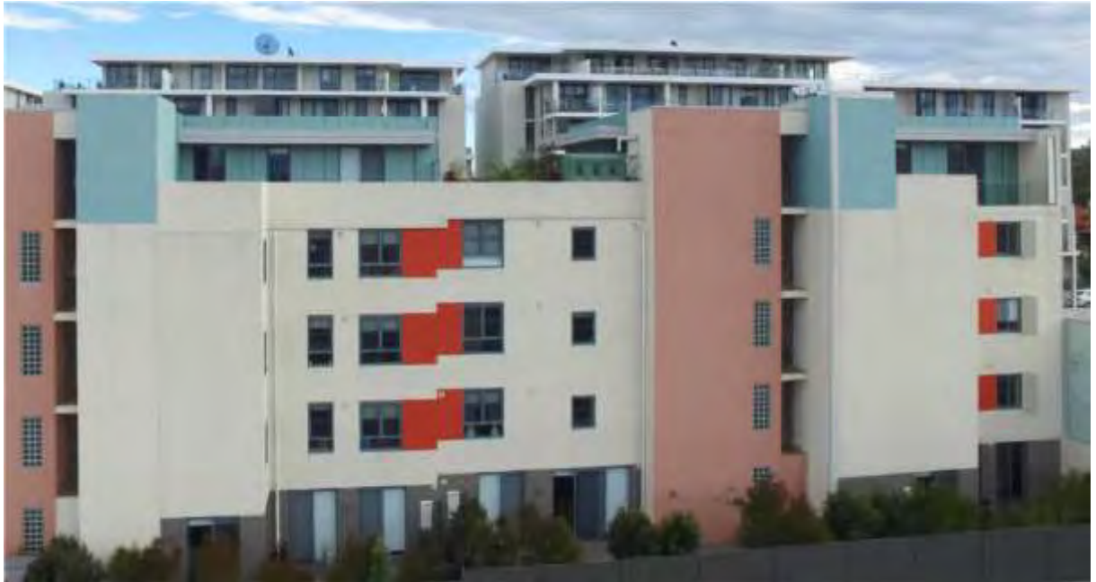
Figure 14: Photograph showing the eastern façade of 4-8 Angas Street. The development at 3-13 Angas Street is located in the background.
