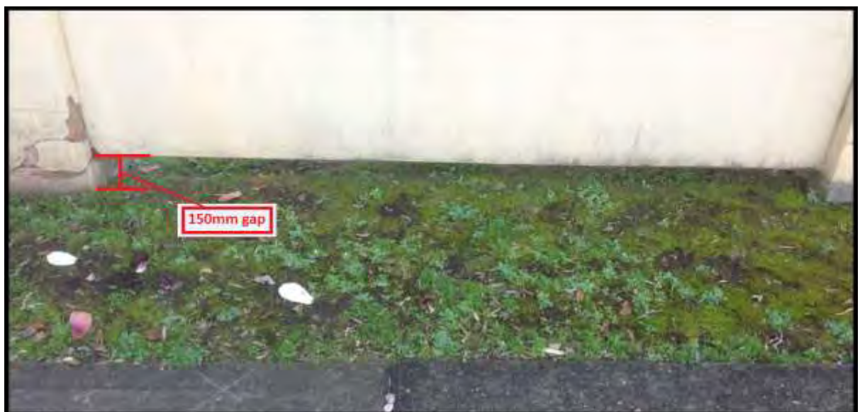
Close-up photo of the left panel with a clearance of 150mm which is the requirement for the front fence in the subject DA.
