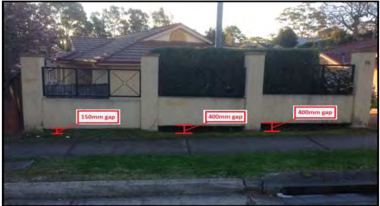
Example of solid fence with clearance at the base to allow for overland flow. Note the centre and right panels have a clearance of 400mm, and the left panel has a clearance of 150mm which is the requirement for the subject DA
