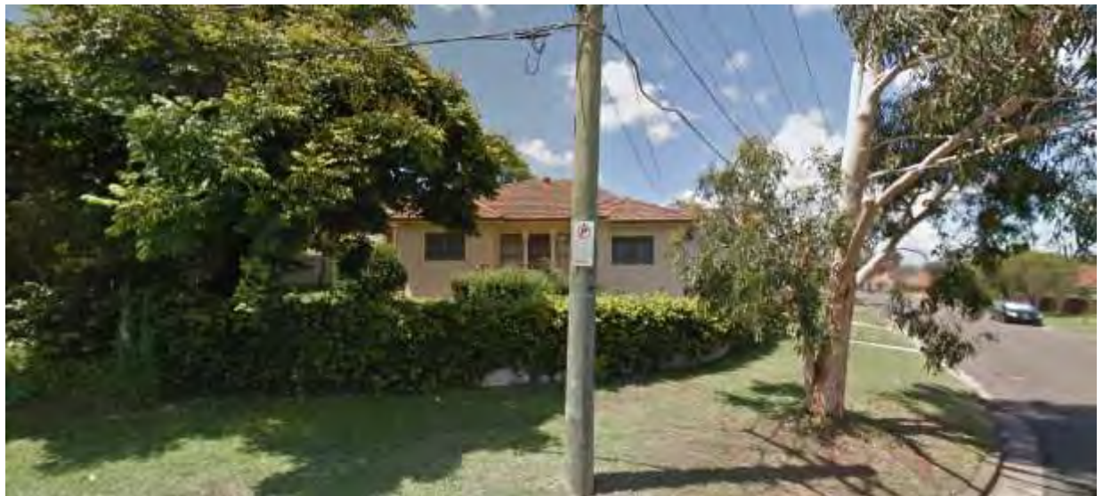
Figure 2a – North west elevation of existing dwelling on site Source: Google Street View
