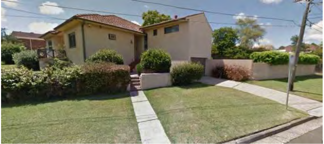
Figure 2b – South west elevation of existing dwelling on site Source: Google Street View
