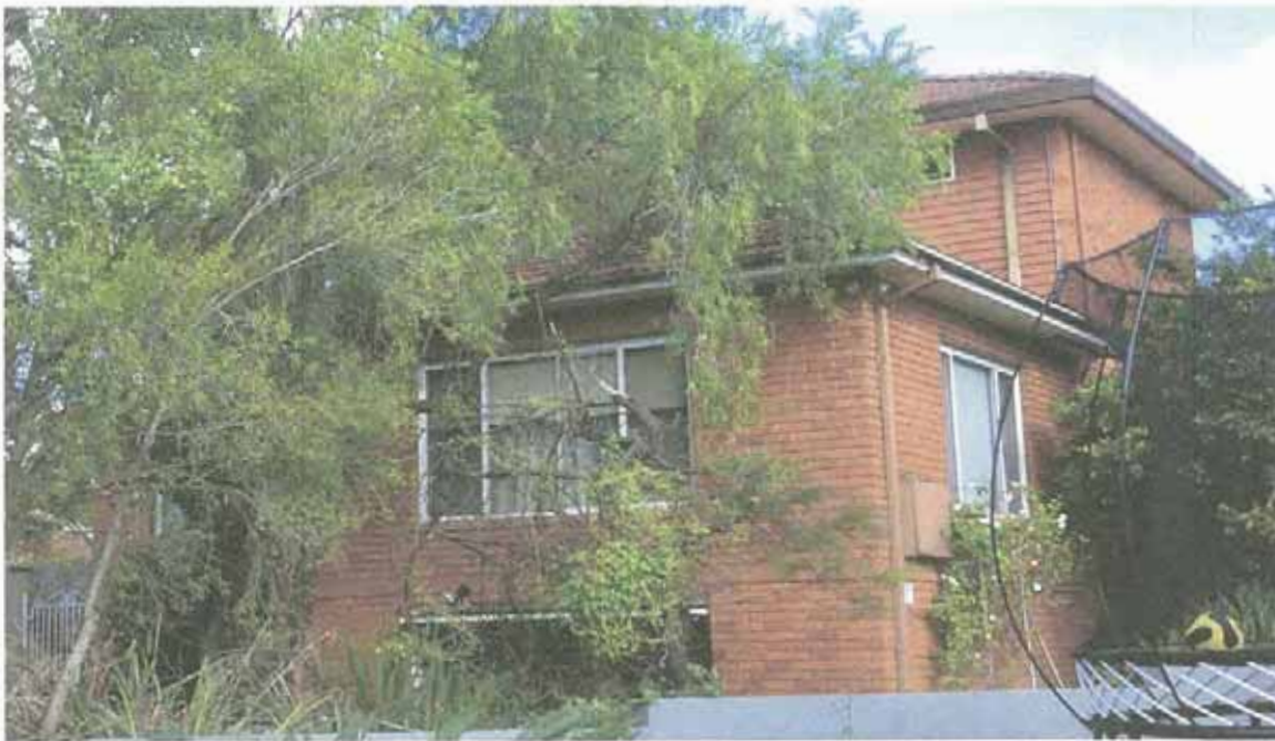
Existing house (manse) at 16 Vera Street Eastwood
