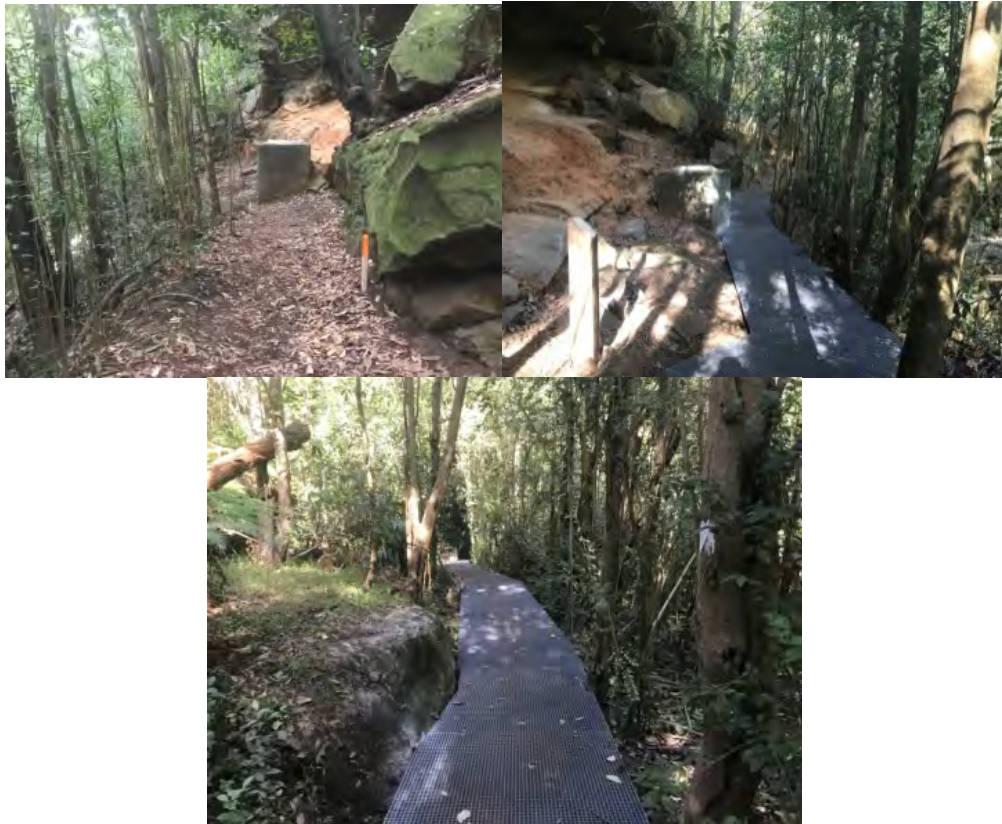
(Before and After - decking installation)
