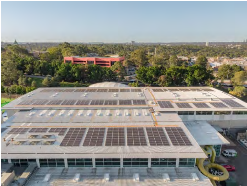
(RALC Solar installation – is to be finalised in November 2018)
