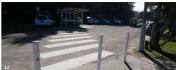
17. The pedestrian crossing from the wharf cuts through the carpark and leads to a disused bus stop now used by persons being dropped of or picked up from the ferry wharf in hot or wet conditions.
