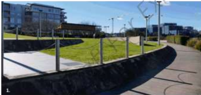
1. Helene Park was created as part of the Shepherds Bay development, connecting the high density residential area to the waterfront.
