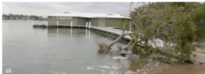
13. The Concord Ryde Sailing Club house is built on timber piers above the high water mark. The Rivercat Ferry wash causes the beach to erode and the mangroves to deteriorate.
