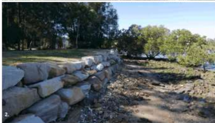
2. A small sandy beach at Memorial Park provides direct access to the river. The sea wall is constructed with sandstone blocks.
