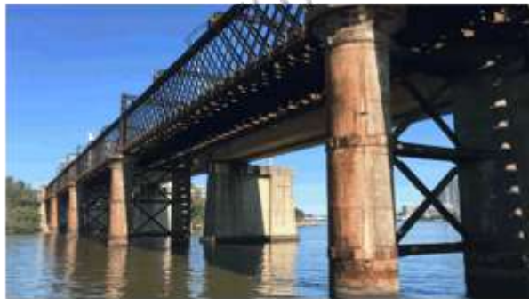
The Ryde Railway Bridge is a double lattice girder bridge that survives substantially in tact. In 1980 it was decommissioned as a rail bridge and is now used for shared access for bikes and pedestrians to link to other walking and cycling trails such as the Parramatta Valley Cycleway. It is listed on the NSW State Heritage Register.
