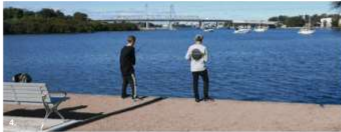
4. The southern part of Anderson Park has open views across the river. The seawall needs upgrading.
