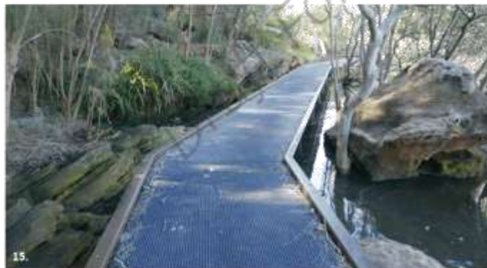
15. A fibreglass mesh boardwalk winds through the mangroves at Glades Bay Park
