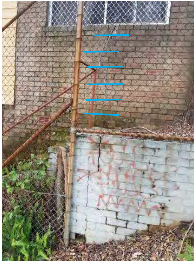
Photo 39 – locations of brick stitching.
