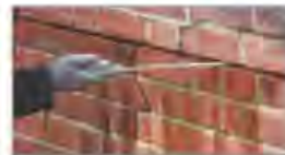
2. Clean out slots and flush with clean water and thoroughly soak the substrate within the slot
