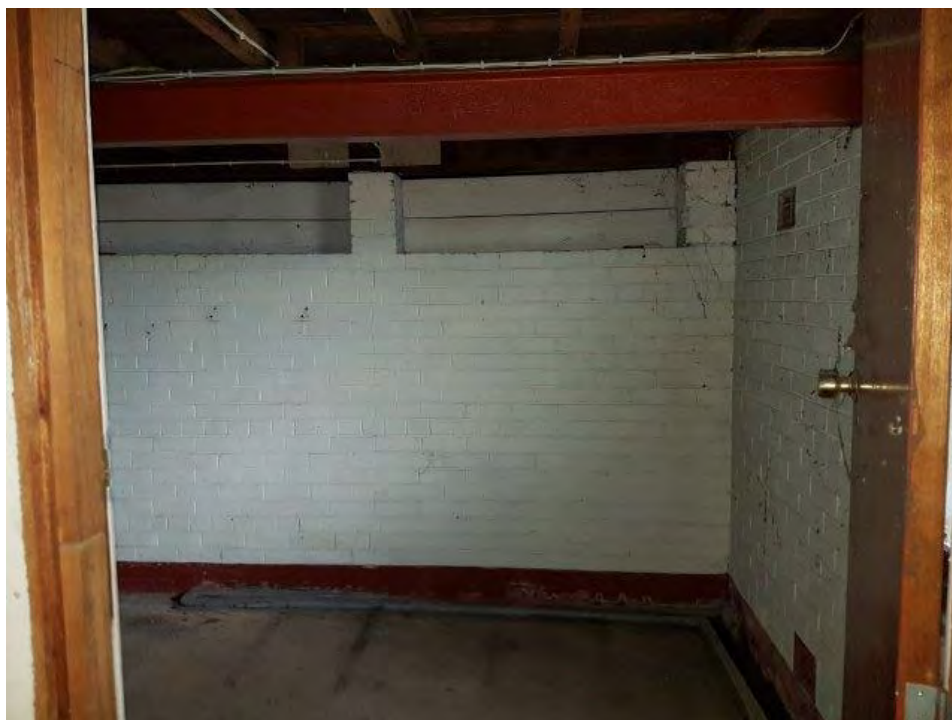
Photo 18 – General condition of basement brick wall & steel beam.
