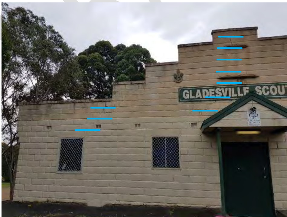
Photo 38 – locations of brick stitching.
