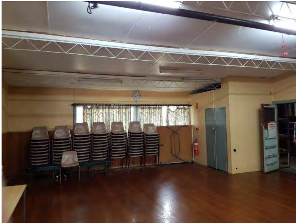
Photo 3 – General condition of internal areas
