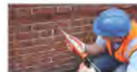
6. Re-point the mortar bed and make good the vertical crack with CrackBond TE
