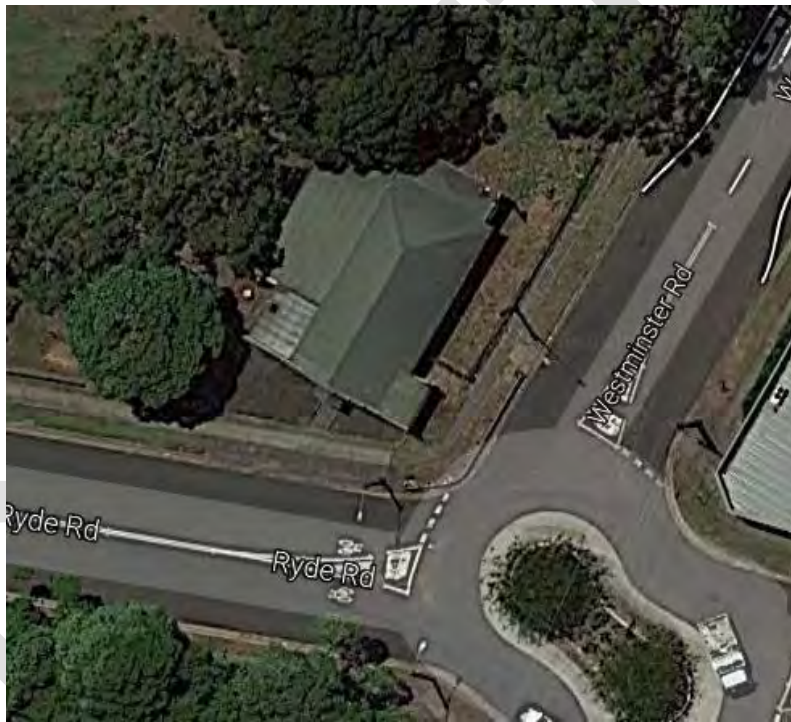
Figure 1: Aerial view of the property
