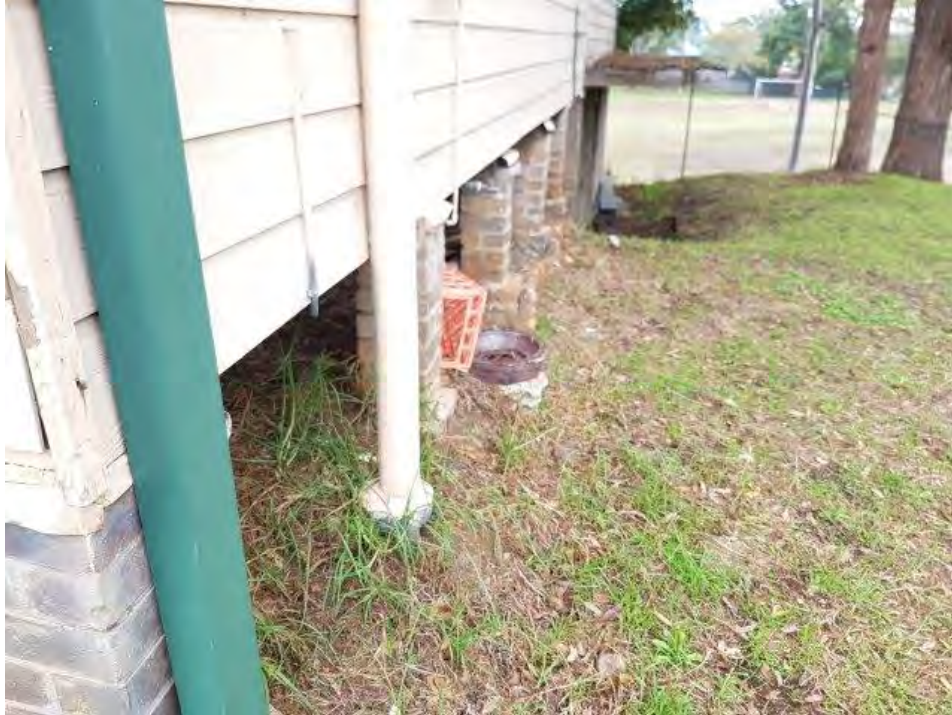
Photo 31 – demolish and rebuilt edge piers.
