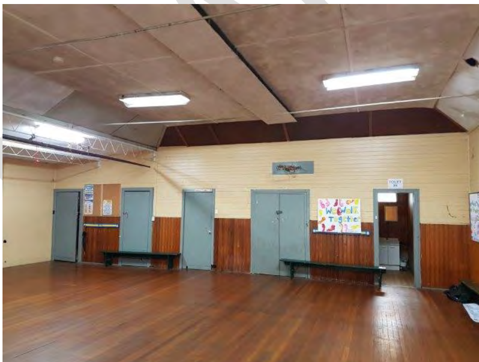
Photo 4 – General condition of internal areas
