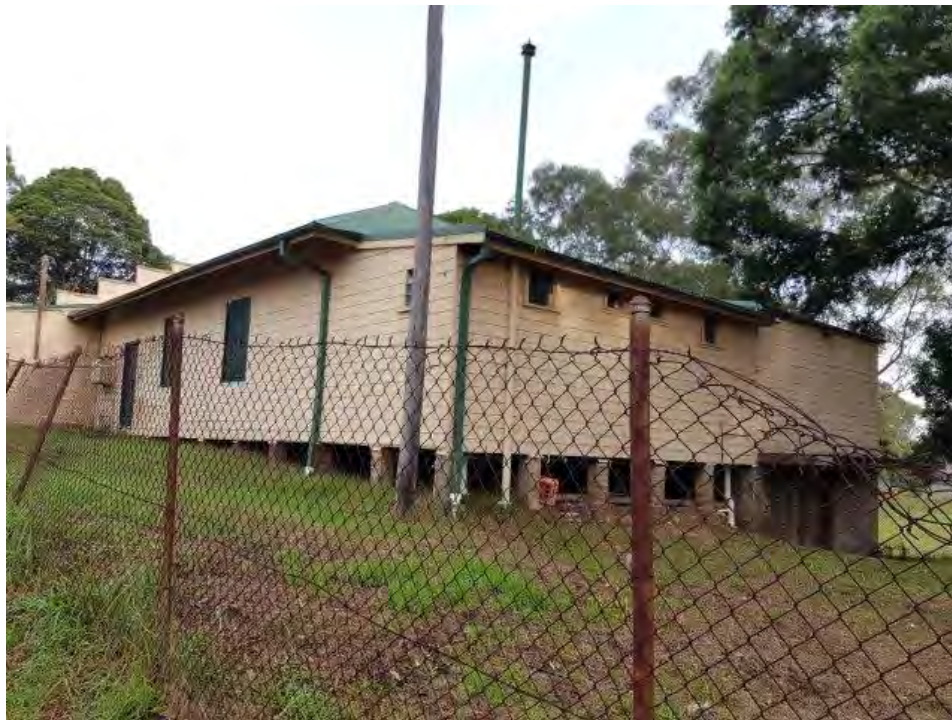
Photo 1 – General condition of the building
