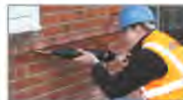
3. Using the Helifix Pointing Gun, inject a bead of HeliBond along the back of the slot
