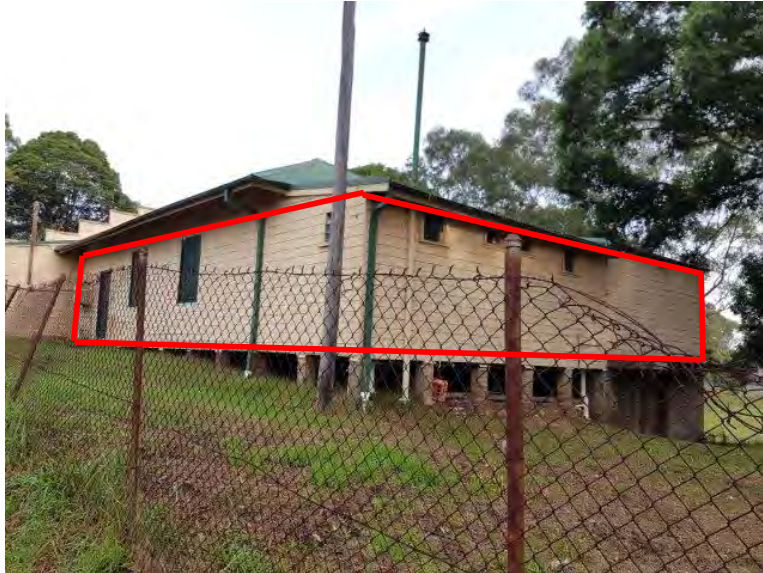
Photo 32 – replace external cladding.
