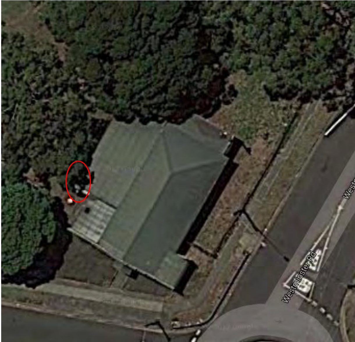
Figure 5 – location of existing retaining wall to be replaced.
