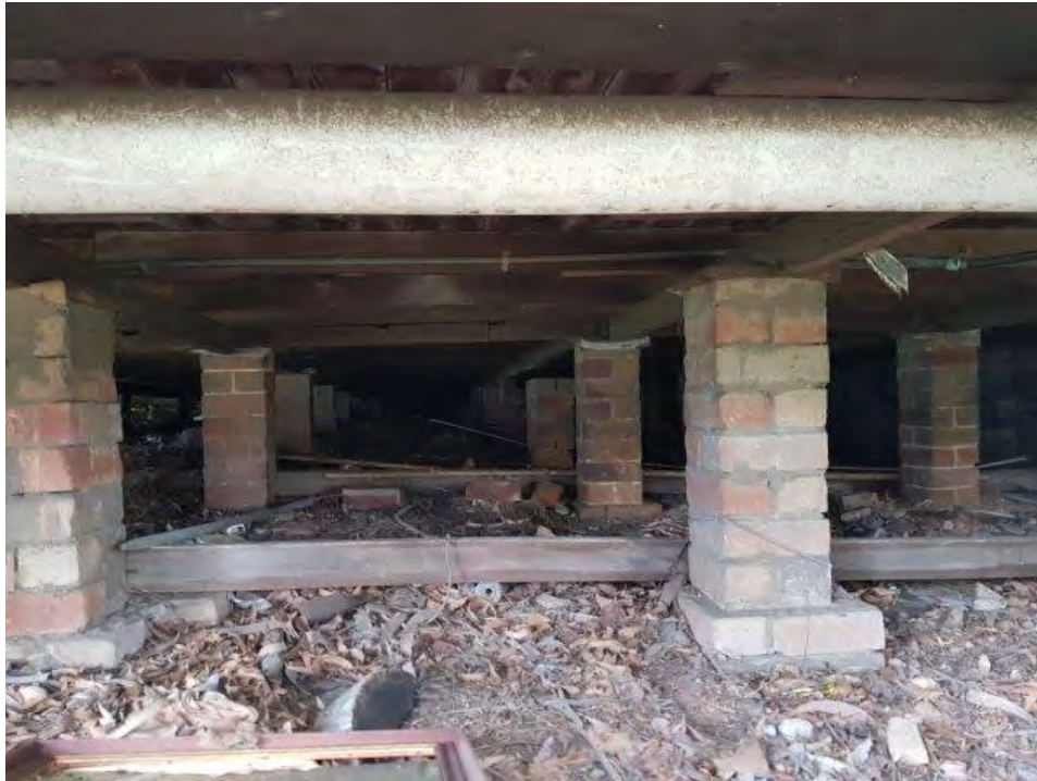
Photo 5 – General condition of existing brick piers
