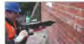
5. Insert a further bead of HeliBond over the exposed HeliBar, finishing 10 – 15mm from the face, and 'iron' firmly into the slot using the HeliBar Finger Trowel
