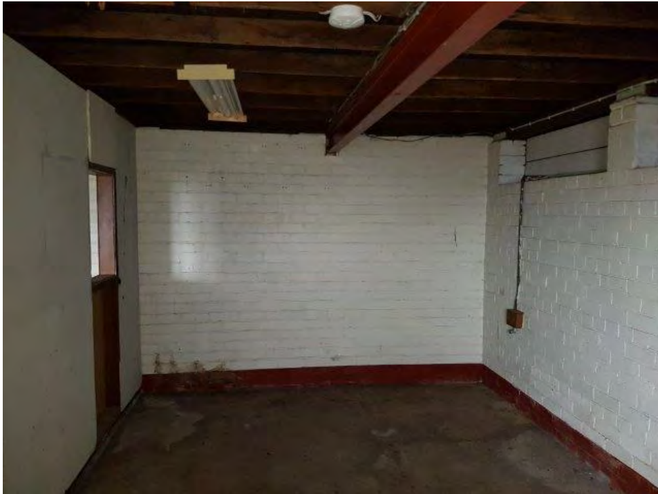
Photo 17 – General condition of basement brick wall & steel beam.
