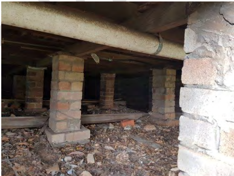
Photo 6 – General condition of existing brick piers
