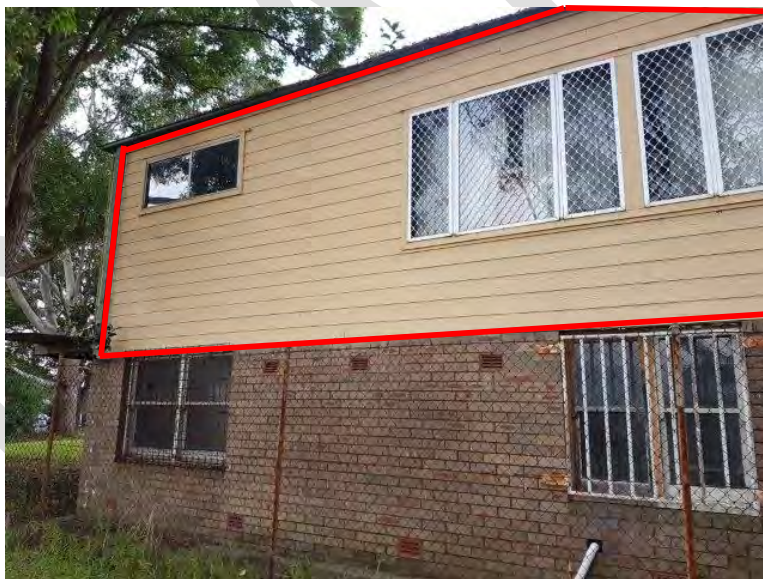
Photo 33 – replace external cladding.
