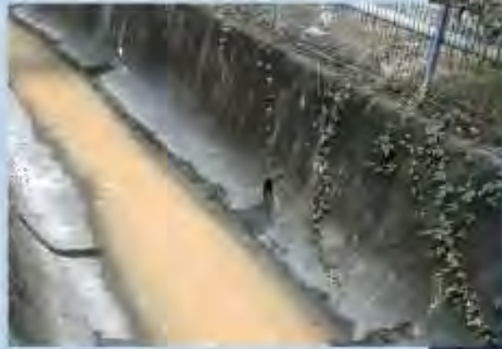
Above: Sediment flows over a weir construction site at Harlow Park. Right: Annotated development of Westcreek from the Parramatta River.
