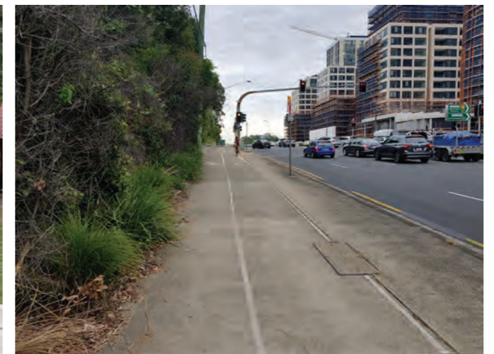
Fast moving cyclists create potential hazard to park users exiting from the park along Epping Road
