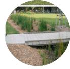
Vegetated swale at the base of the southern embankment to assist with the management of some of the overland flow.
