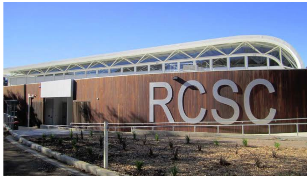
Figure 26: Ryde Community Sports Centre (Photo: YMCA)
