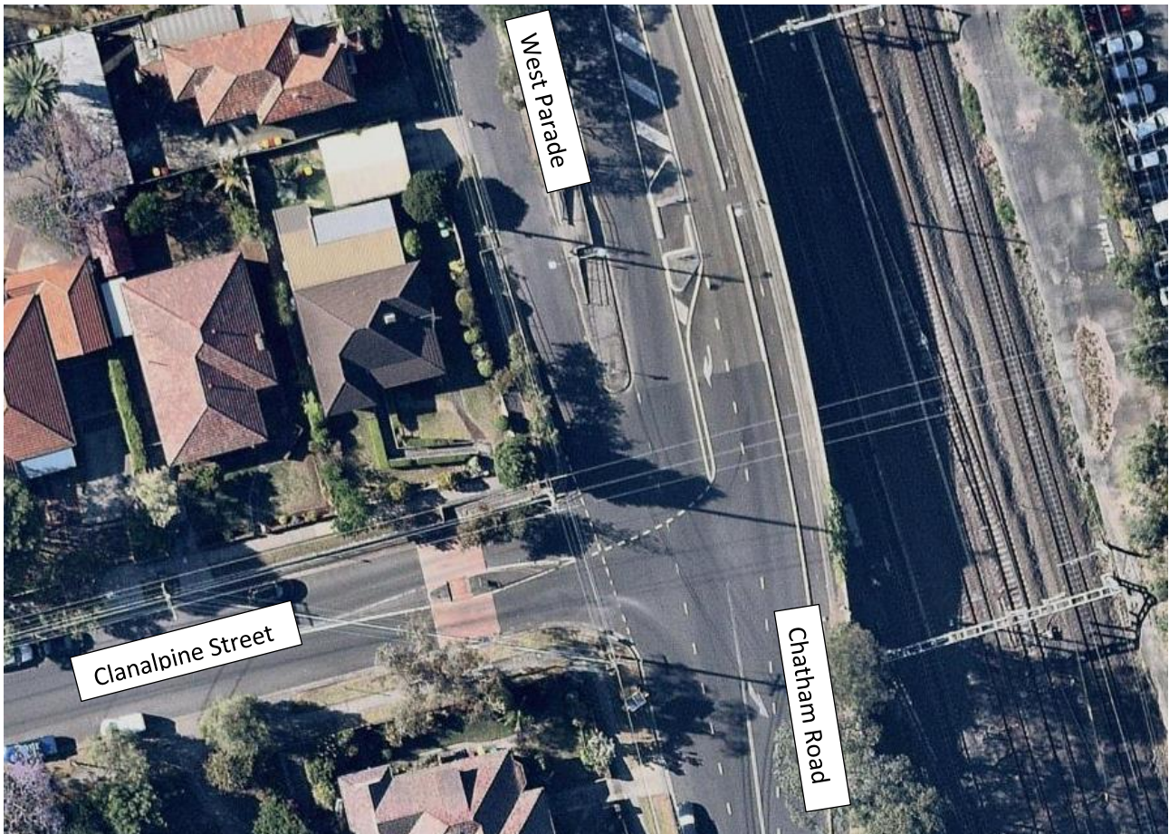
Figure 17: Intersection of West Parade/Chatham Road/Clanalpine Street
