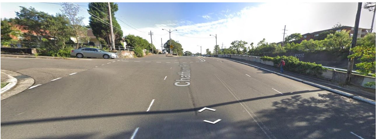
Figure 19: Street view – Looking North at the Subject Intersection
