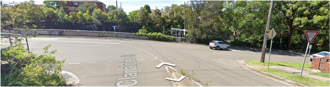
Figure 20: Street view – Looking East from Clanalpine Street
