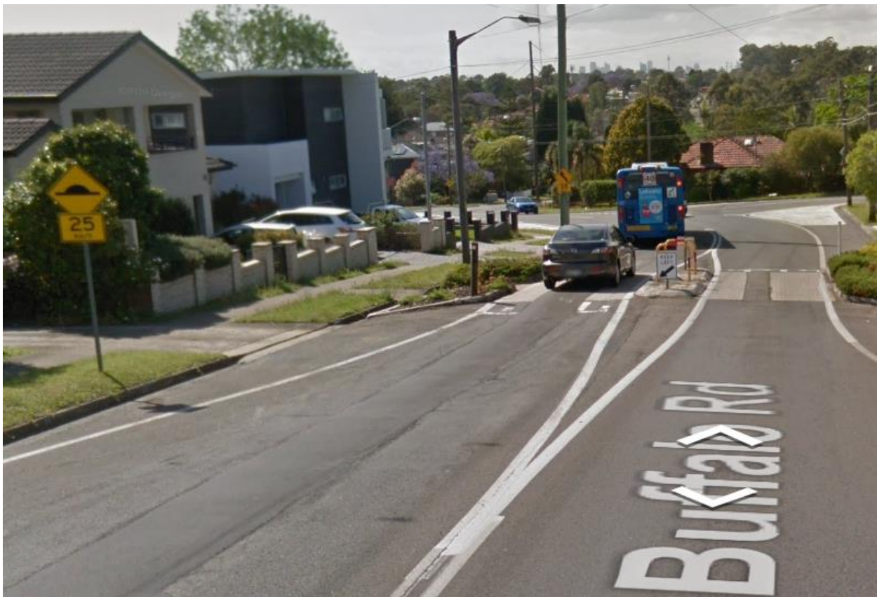
Figure C2: Existing traffic calming facilities on Buffalo Road preceding Aitchandar Road
