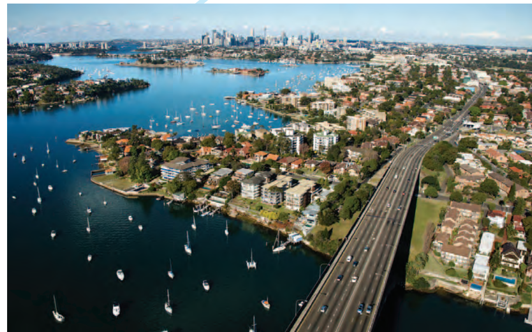
Gladesville Bridge, Victoria Rd, Drummoyne
