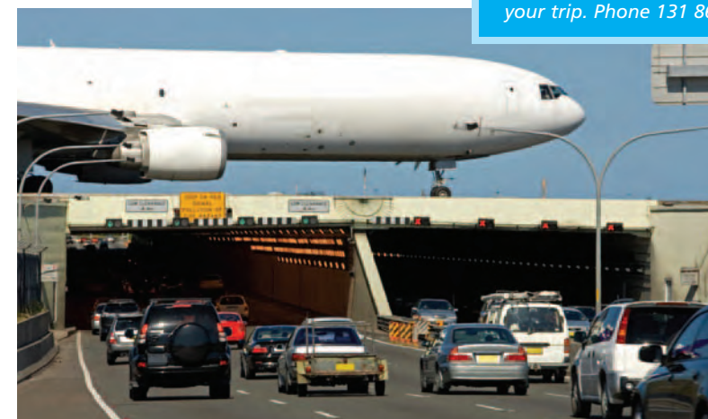
Sydney Airport Tunnel
