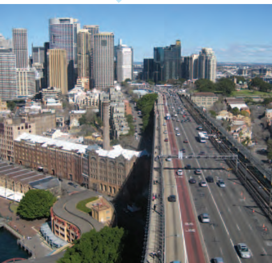
Bradfield Highway on approach to Cahill Expressway
