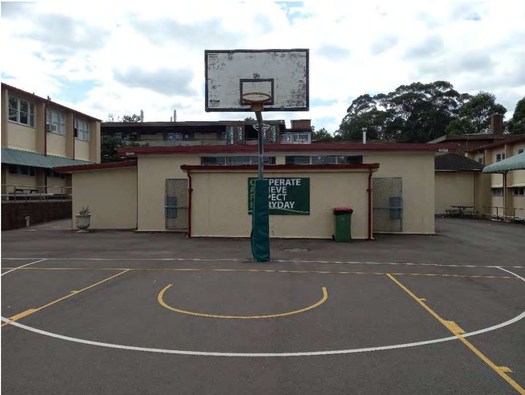
Figure 17 Existing built form
