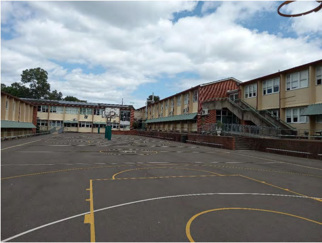
Figure 18 Existing built form
