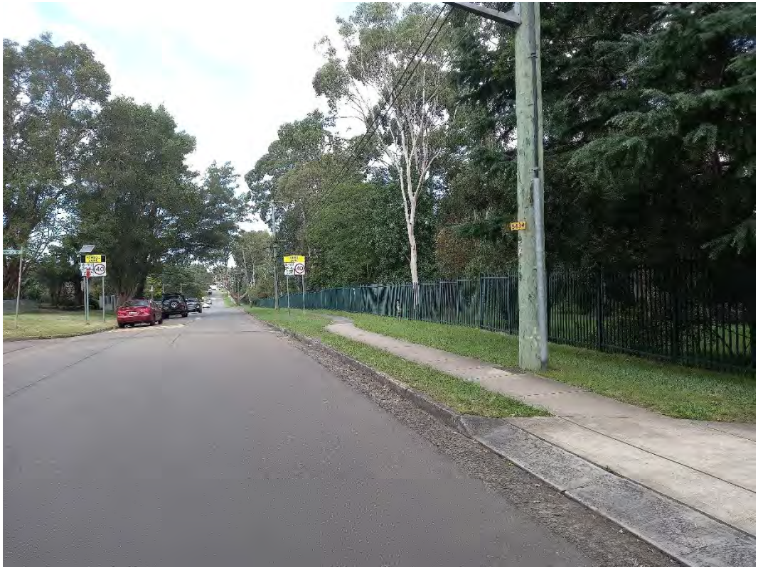
Figure 22 Brush Road looking south
