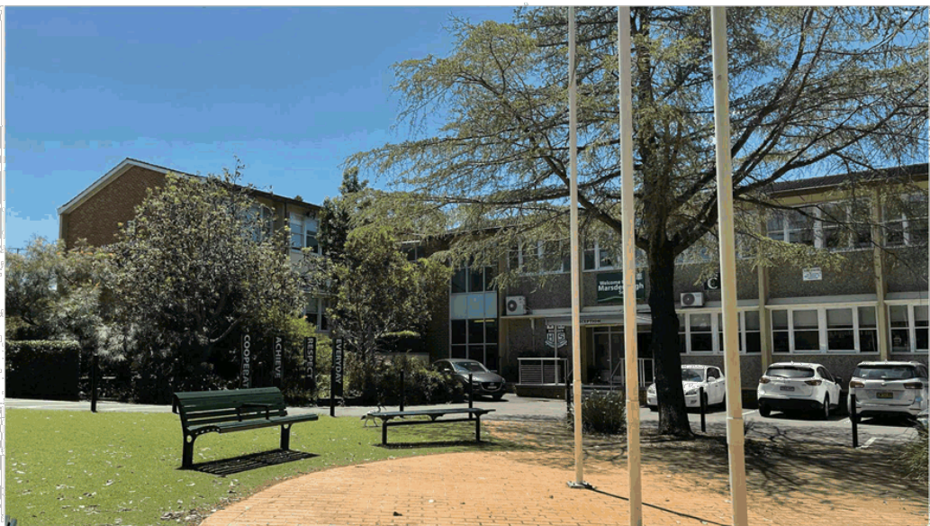
Similar Current view of the main entrance to Marsden High School, Buildings B00B (left) and B00C (right).
