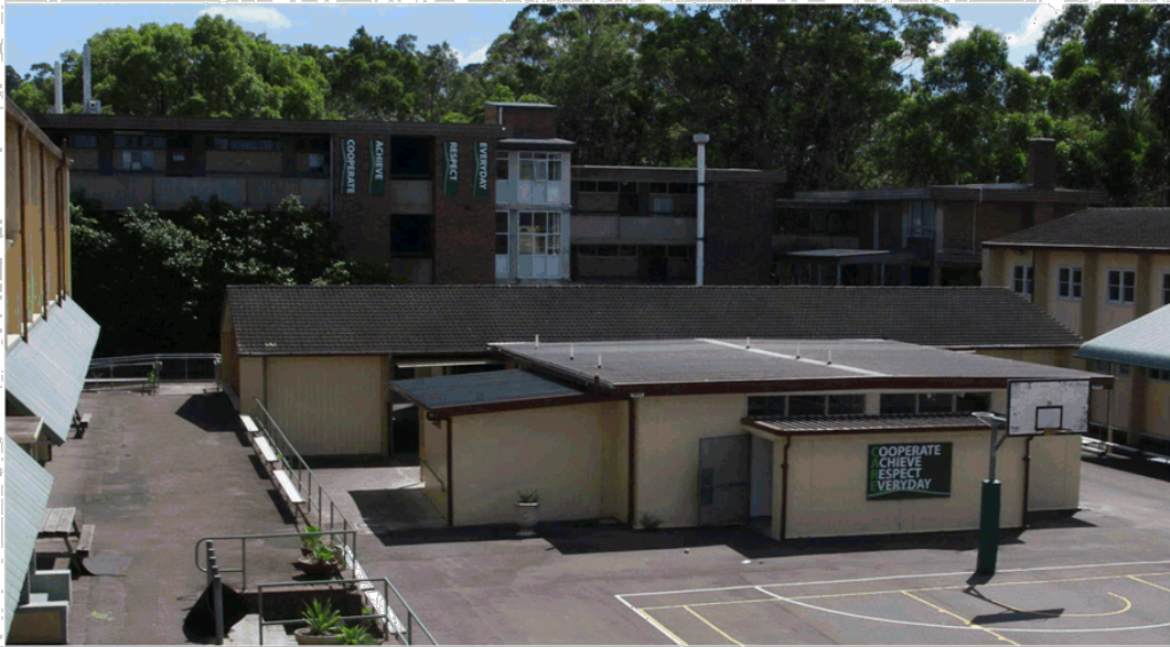
Pupil Facilities and Food Services Unit (Building B001 - formerly G, Stage 1) with the 1971 additions behind: Buildings B00H - right, B00J - centre and B00K - left.
