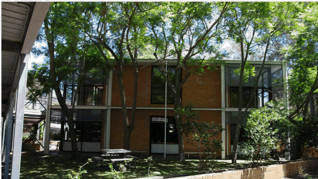
The Library (Building B00G) with the covered walkways connecting it to Buildings B00A and B00K.
