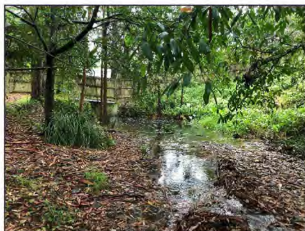
Photograph 6: View north to culvert at top of creek line
