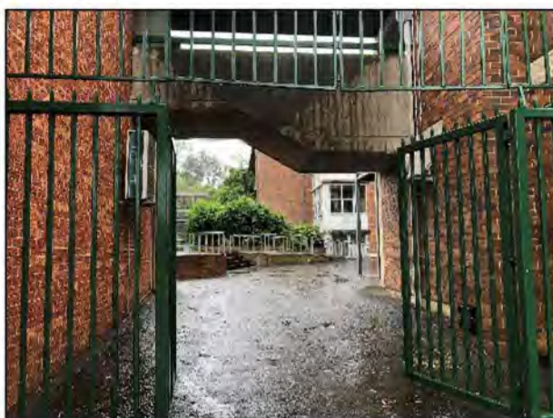
Photograph 1: View north west into school buildings
