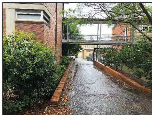
Photograph 4: View north west into school buildings
