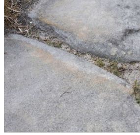
Track features - stormwater management using a drain cut into insitu rock.
