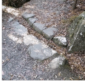
Track features - stormwater management using a stone gutter / box drain.
