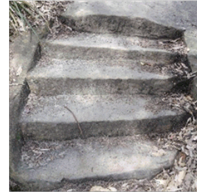
Track features - steps cut into insitu rock.
