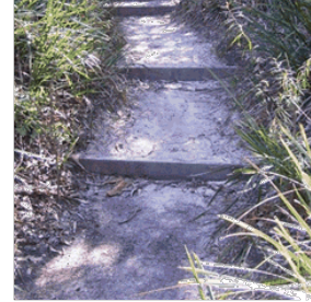
Track features - sleeper step and runs with sand or compacted fill treads.
