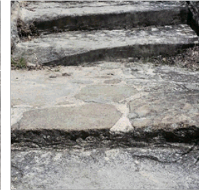
Track features - infill stone flagging and rock leveling to create a passable track over insitu rock outcrops.
