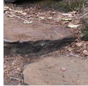
Track features - landing tread stone to armour track and prevent wearing from use.
