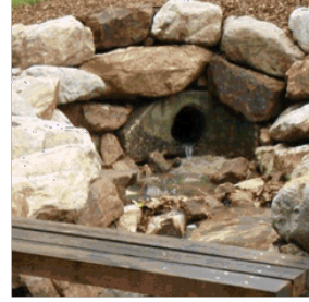
Rock lined headwalls and drainage lines to stormwater water outlets to manage erosion, before flowing to planted bio swales.
