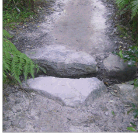
Track features - rock lined box drain / gutter.
