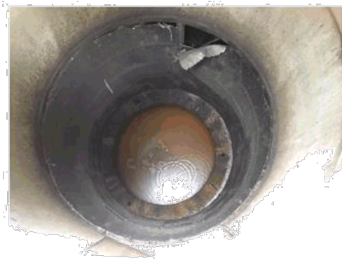
Looking inside the device. Note this photo was taken in May 2018 and shows the former damaged screen that Optimal Stormwater repaired for TDC for Ryde Council in 2018.
