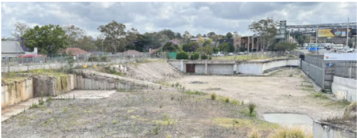
Figure 1 - Photo showing the basement of the former council building that is proposed to be filled.
