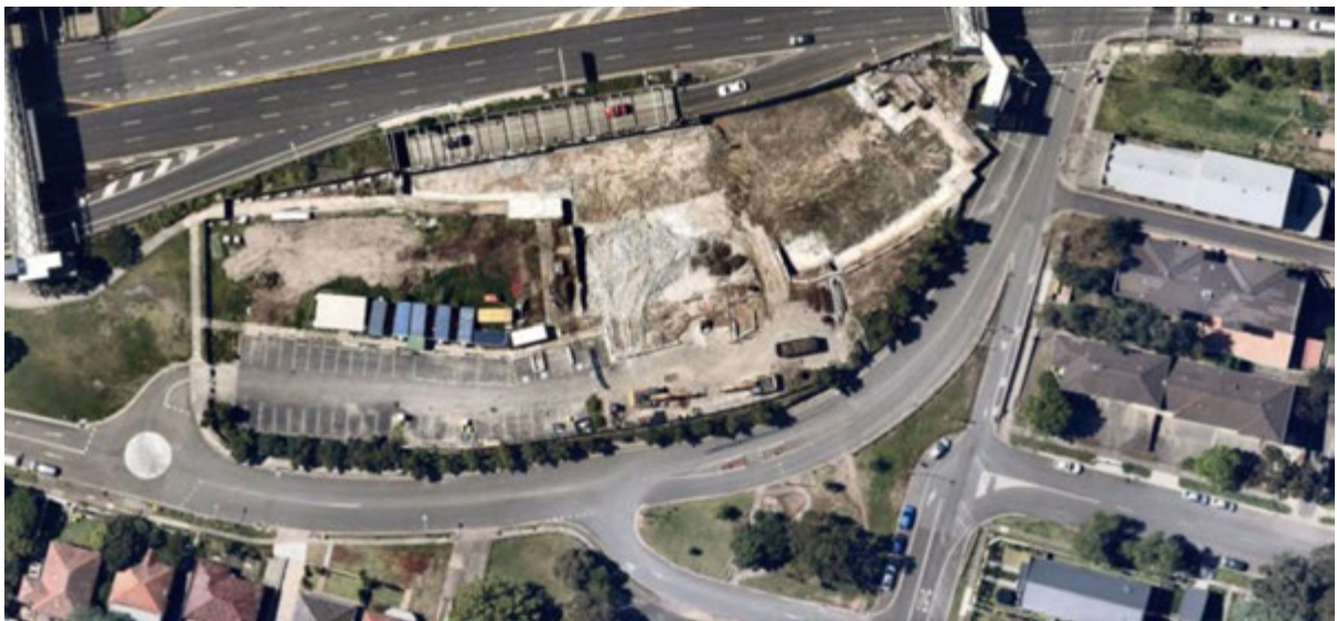
Figure 2 - Aerial photo of Ryde Central dated 4 October 2021.
