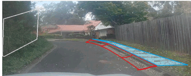
Figure 18: Chainage 40-60 showing the recommended rolltop kerb in red, the hard stand area for kerb-straddle parking in teal, and the tree pruning works in white.
