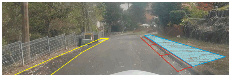
Figure 26: Chainage 300-330. There is more opportunity to recommence rolltop kerbs (red) in this section due to the more level verges. A parking hard stand can also be provided to allow vehicles to straddle the kerb when parked (teal shaded area). The full-depth pavement reconstruction should continue as per the yellow polygon.
