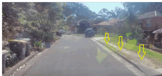
Figure 5: At chainage 80, there is a pronounced "scar" along the turfed council strip where the right-wheels of parked cars track and rest when vehicles are straddled on the kerblines when parked. This indicates the frequency and the necessity of this practice to make the roadway pass-able and operational. View from inside the truck.
