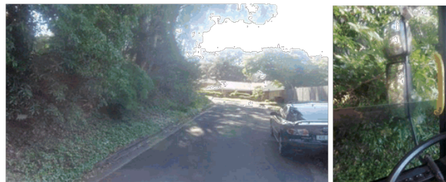
Figure 4: Between chainage 20-60, there is a risk of the waste collection truck scraping/ impacting the roadside vegetation. Much of this vegetation encroaches over the plumb line to the kerb and is therefore an obstruction hazard. Note also the lack of passing clearance, particularly if the parked vehicle was positioned wholly in the roadway instead of being straddled across the kerblines. Note the tyre marks along the left-hand kerb indicating frequent wheel strikes. The right-hand photo shows the wing mirror of the truck impacting the overhanging tree foliage. Views from inside the truck.
