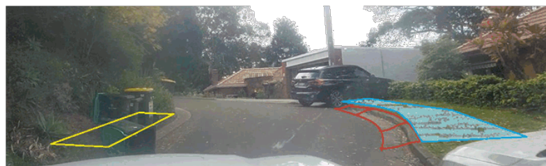
Figure 21: At chainage 170, by providing rolltop kerbs (red) and parking hard stand areas (teal), it is hoped that vehicles will not park in driveways as shown. This should free up more space for the truck to complete the 180° hairpin turn.
