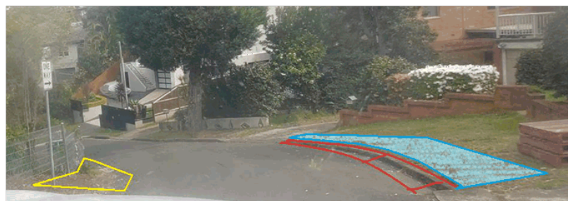
Figure 27: Chainage 330. The recommended rolltop kerb and pavement hard stand area (red and teal shaded areas) would greatly improve access and width for trucks turning at this point. The full-depth pavement reconstruction could continue in the yellow section.
