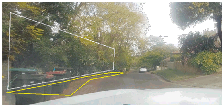
Figure 22: Chainage 195-200 – the commencement of the higher elevation section of Buena Vista Avenue. The strategy changes to providing more full-depth pavement along the left-hand side of the route (yellow polygon), repairs to the fencing and tree pruning works (white polygon).
