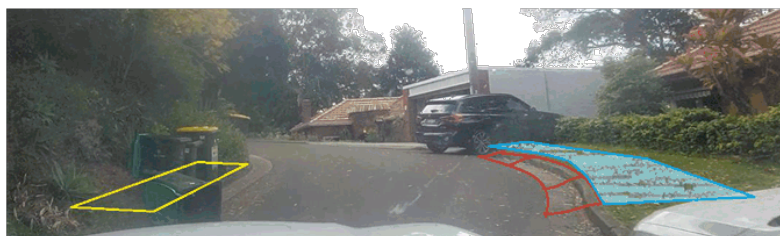
Figure 21: At chainage 170, by providing roltop kerbs (red) and parking hard stand areas (teal), it is hoped that vehicles will not park in driveways as shown. This should free up more space for the truck to complete the 180° hairpin turn.
