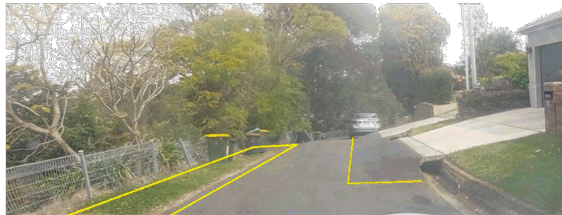
Figure 24: Chainage 246. There is less opportunity for rolltop kerbs since the verges are steep and some even contain retaining walls. The full-depth pavement widening and fence repairs should be carried out on the left-hand side of the road (yellow). Bases of driveway ramps should be outlined in orange. Note the fence which also requires repair work.
