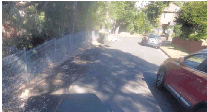
Figure 12: At chainage 300, an example of an extended pavement area on the left-hand side of the roadway. This is not a deep lift. Rather, the pavement extension is only on the surface. The load-bearing capacity of this extended asphalt strip is questionable.
