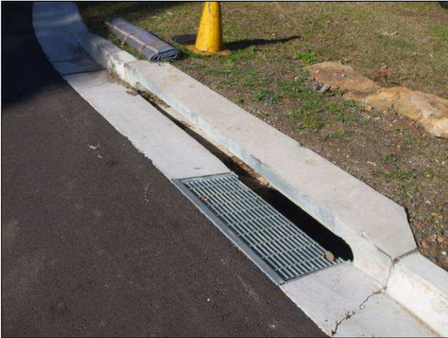
Photo 13: Sewer entrance on Field of Mars Reserve, looking south.
