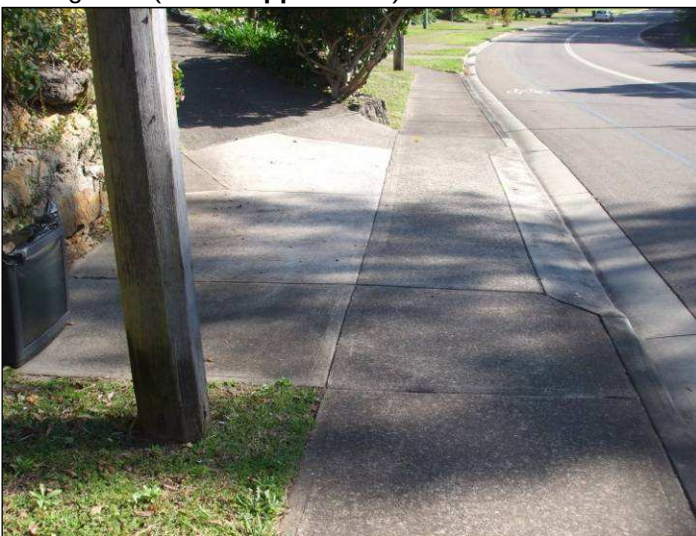
Photo 17: View of driveways to be re-aligned, looking north.
