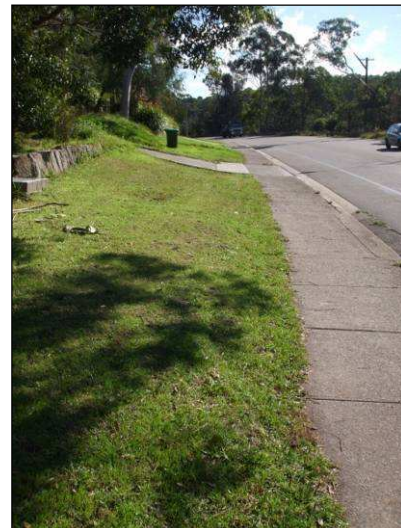
Photo 16: Example of sections of existing footpath to be demolished.
