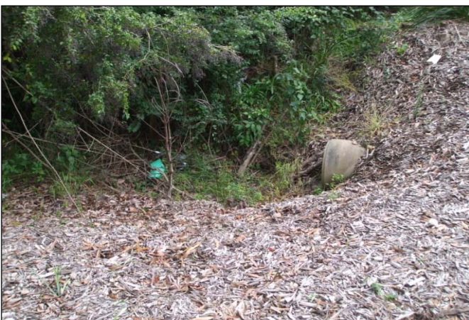
Photo 23: Drainage outlet to become GPT (Plan 15 Appendix C).
