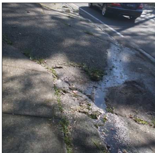
Photo 9: Example of water run-off, looking north on Pittwater Road.
