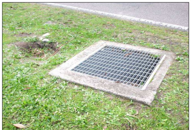
Photo 24: Existing stormwater grate to be removed (Plan 15 Appendix C).
