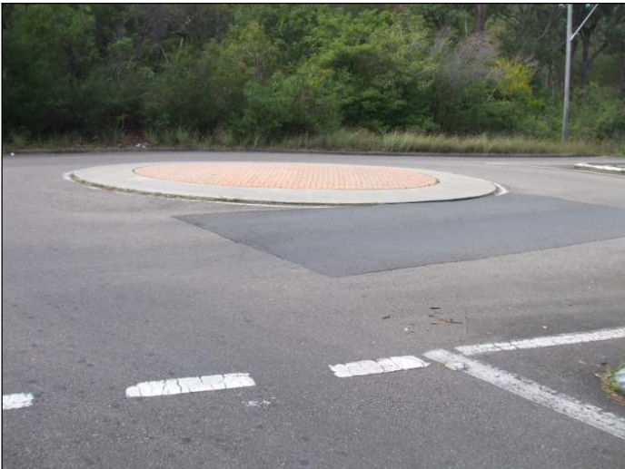
Photo 21: Roundabout at Cox's Road intersection, looking east.
