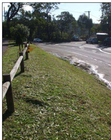
Photo 7: Part of existing rock face to be excavated, looking south along Pittwater Road (Plans 2 and 3 Appendix C ).
