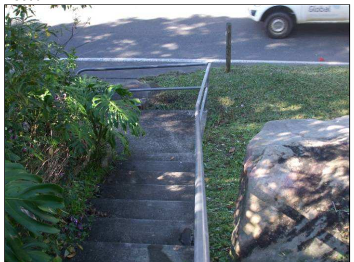
Photo 6: Stairs to be retained and connected to the SUP (Plan 2 Appendix C ).
