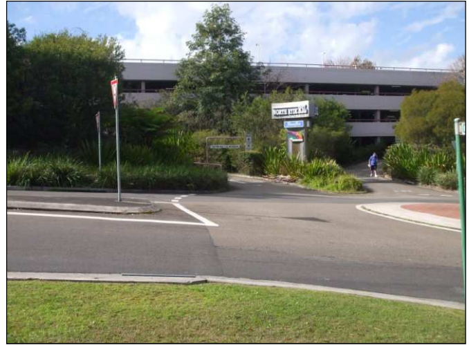
Photo 26: Looking east at Ryde RSL (Carramar Ave roundabout).
