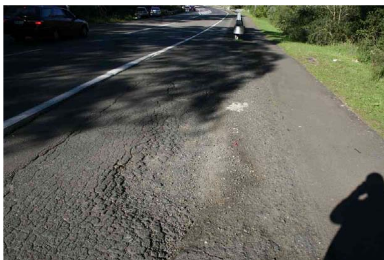
Figure 2.2: Example of an unsafe edge break.
