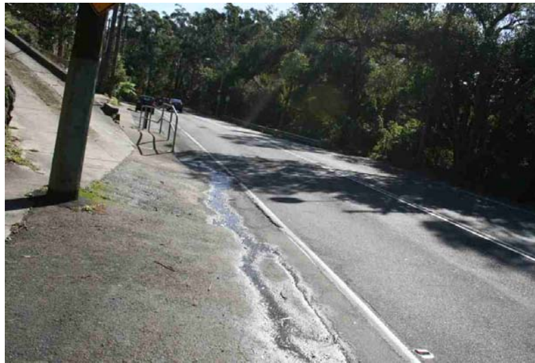
Figure 2.3: Example of irregular road surface.
