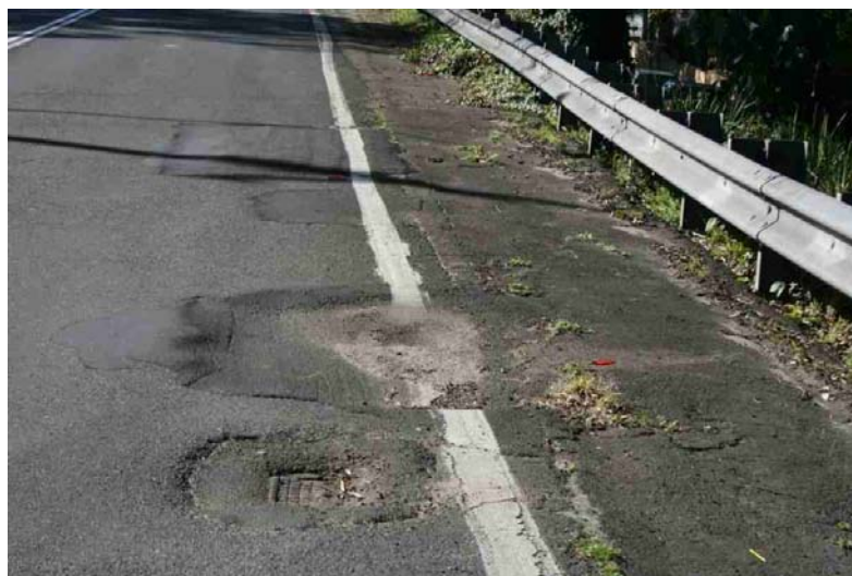
Figure 2.1: Example of failing pavement.
