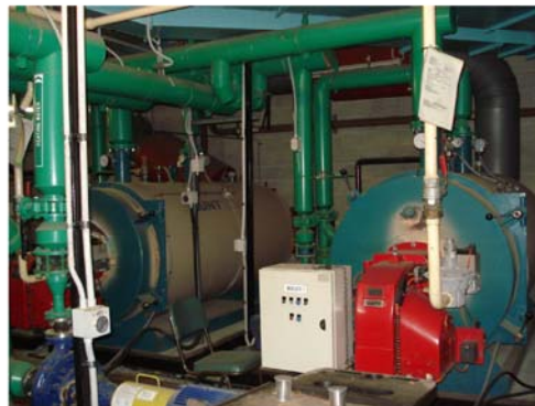
Photograph 1.2 CHP heat recovery to be piped in series with the existing RALC Boiler plant (shown below)
