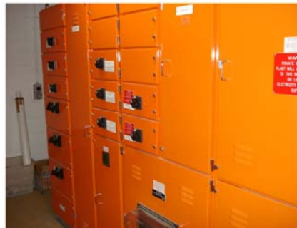
Photograph 1.4 CHP circuit breaker to be installed in RALC Main Switchboard (shown below)
