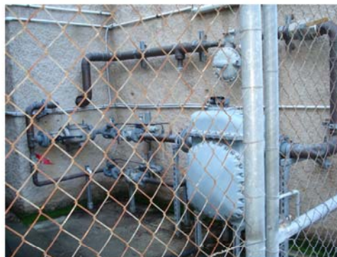
Photograph 1.3 Gas supply for CHP to be tapped from the RALC Main Gas meter and regulator (shown below)
