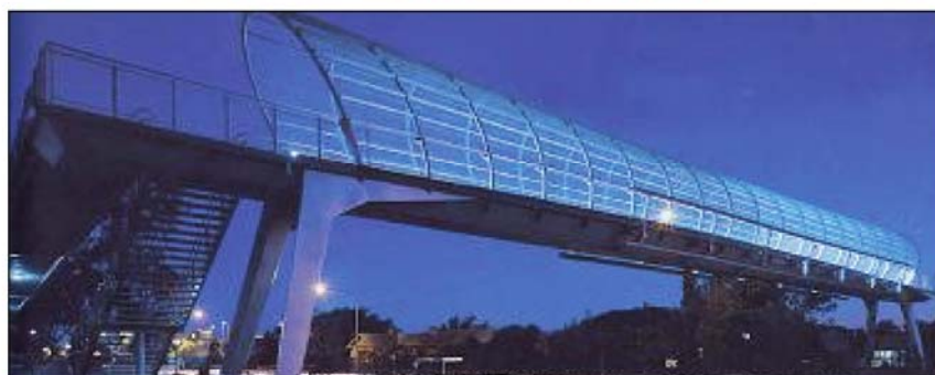
Figure 4.4.23 An example of design excellence: a footbridge designed by Ed Lippman, joint winner of a design competition sponsored by the RTA and NSW Government Architect.
