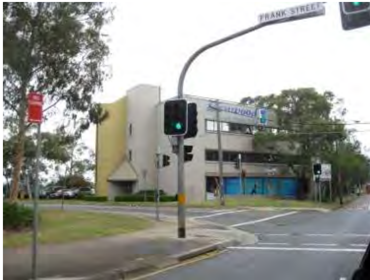
View of 495 Victoria Road – Building H
