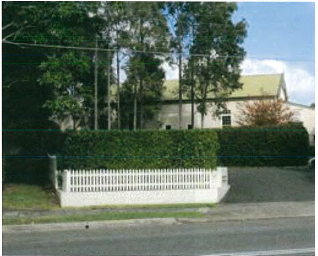
Figure 16 Photograph of the Drill Hall taken from the north looking through the grounds of the town house development to the north, and west of the Drill Hall.
