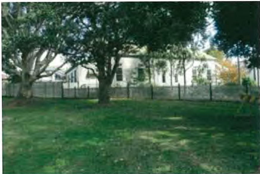
Figure 15 Photograph of the Drill Hall taken from the north in Gladesville Monash Park.
