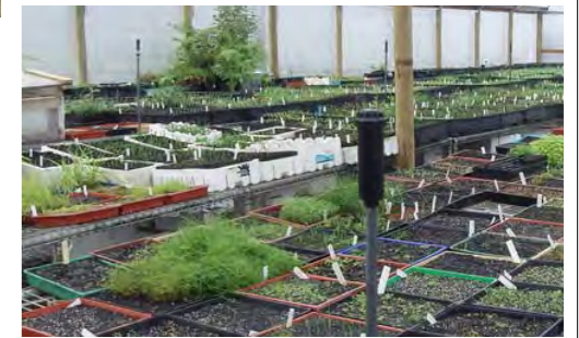
Lightweight Greenhouse Structure
