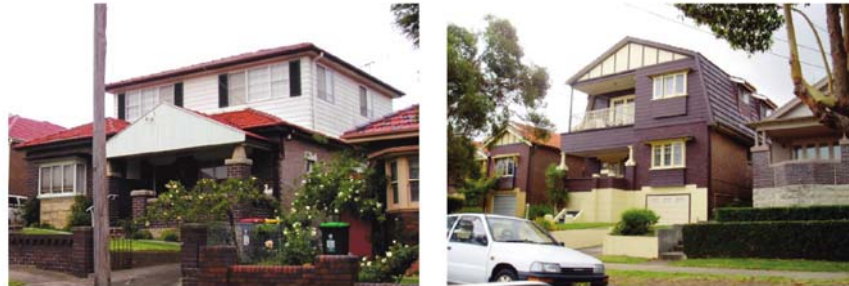
Figure 3.3.02 Examples of unsympathetic alterations and additions.
