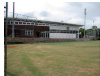
ELS Hall Park with the new indoor sport facility. There is a lack of integration with adjoining sports fields on two sides of the building
