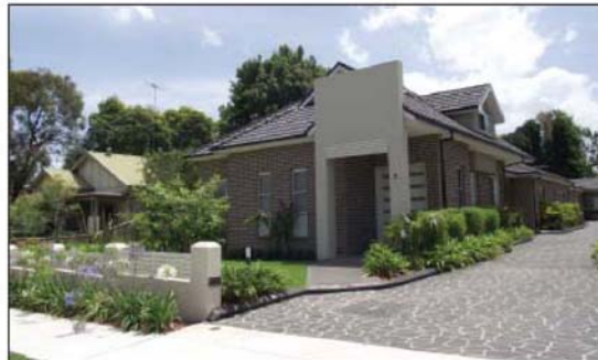
Figure 3.4.3 Villa development with good street address
