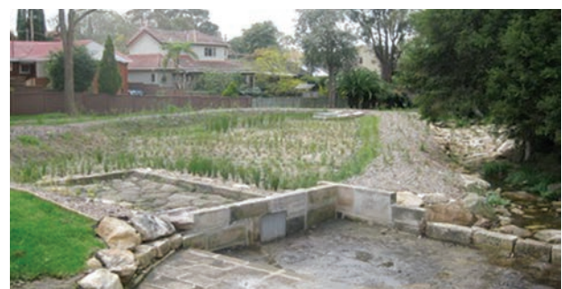
The completed bio-retention basin.
