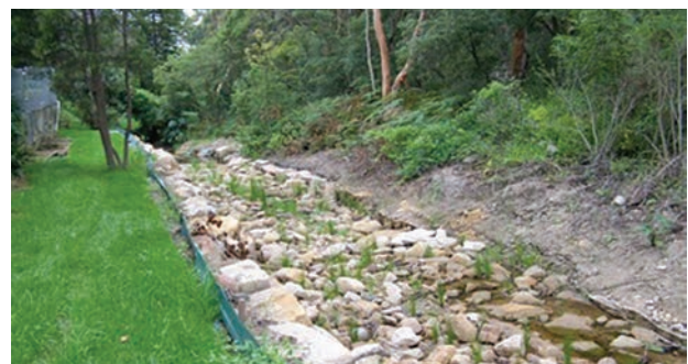
The rehabilitated creek with vegetation starting to grow.
