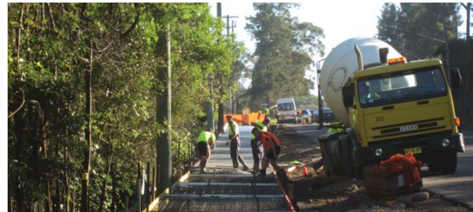
Pittwater Road works.
