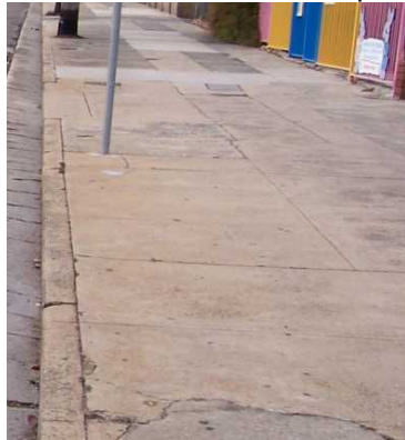
4 – damaged, lifting, major cracking, trips
