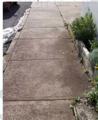
3 – noticeable cracks, uneven, no trips
