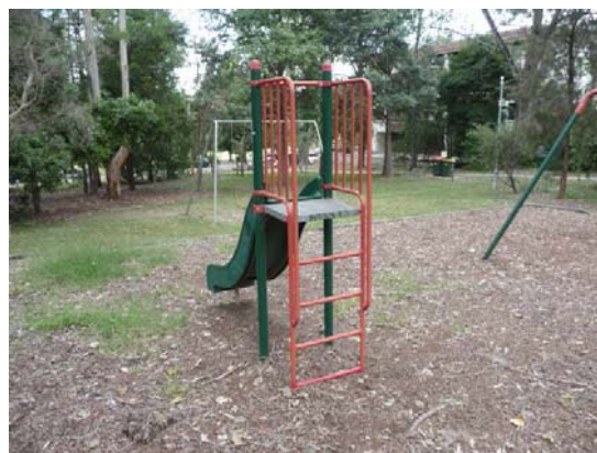
Aging, uninspiring equipment in poorly maintained soft fall material area. This equipment has passed use by date and has outgrown the original demographics which initiated its construction.
