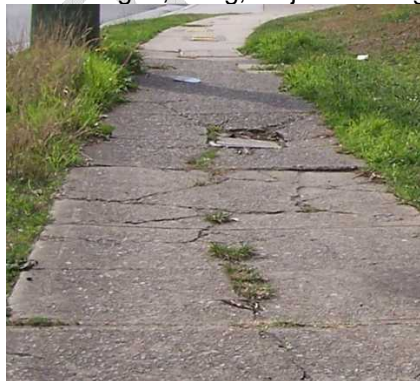
4 – damaged, lifting, major cracking, trips
