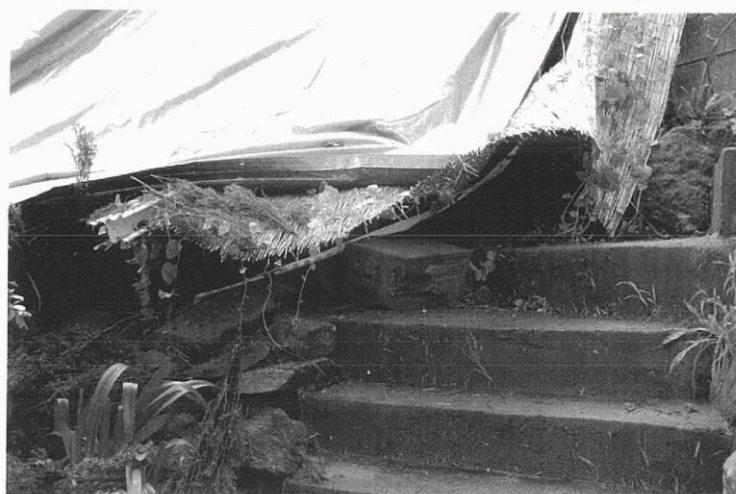
Photo 2 – Edge of slide, displaced piece of retaining wall visible
