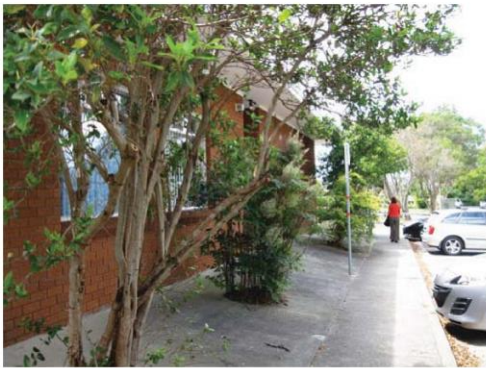
Moncrieff Drive frontage - footpath to be widened and street trees planted. A raised garden bed and new landscaping to be implemented
