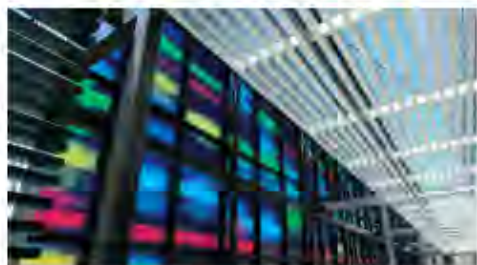
Figure 5.10.3 Police headquarters Parramatta. Here public art is incorporated into the building façade and sunscreens. The art work is based on forensic science and DNA graphs.
