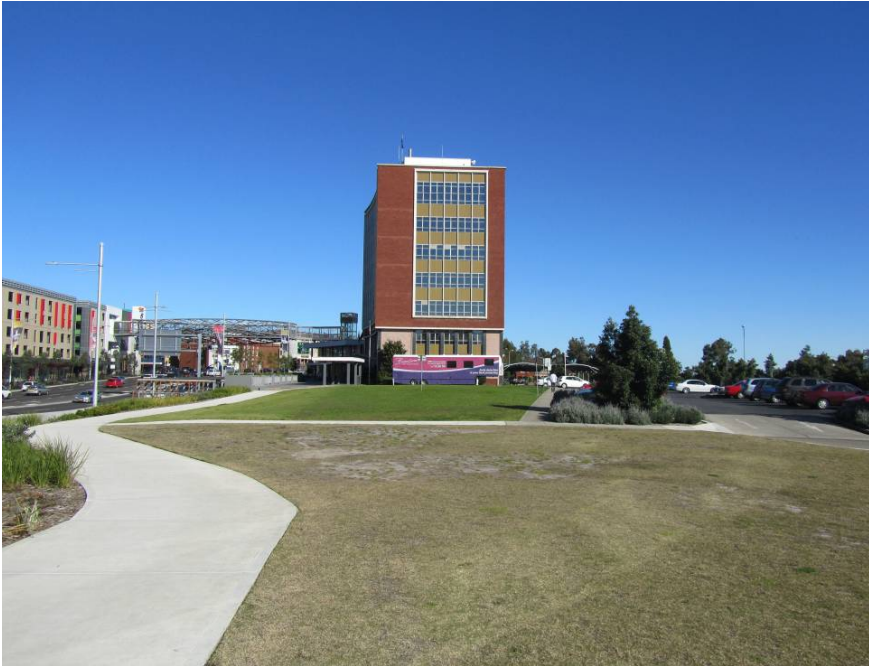
Figure 4 Photograph of existing site and improvements
