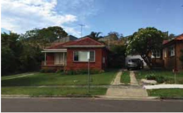
Figure 9: Adjoining dwellings in Brereton Street looking north (Source: Michael Woodland 2013)
