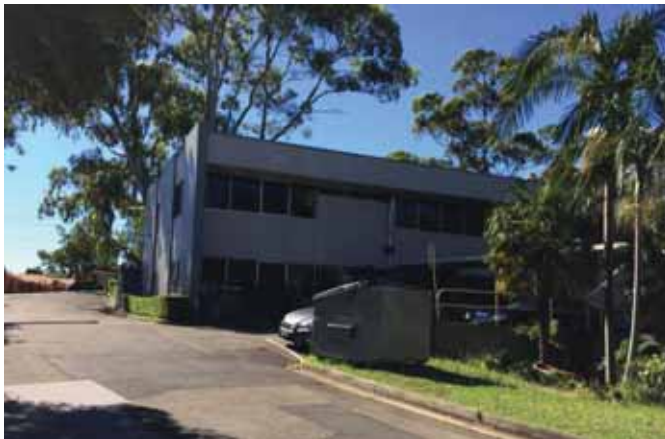
Figure 5: Rear of 2 storey office building on Site A (Source: Michael Woodland 2013)
