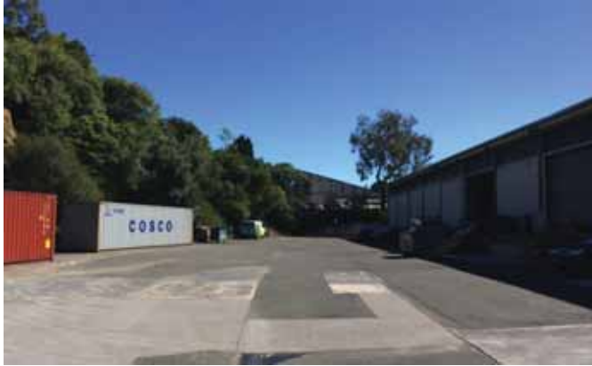
Figure 4: Existing warehouse located on Site A looking south (Source: Michael Woodland 2013)
