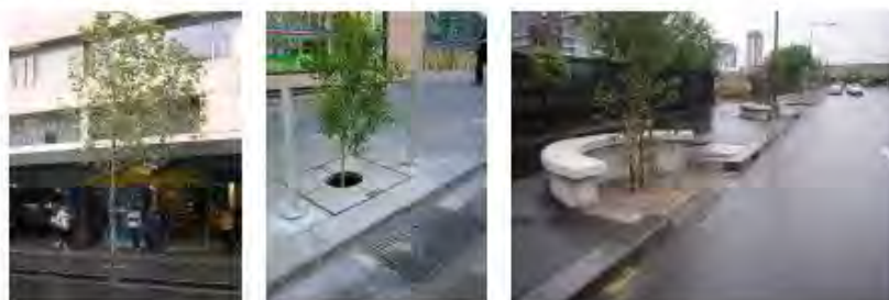
Figure 17 - Example street tree bioretention systems
