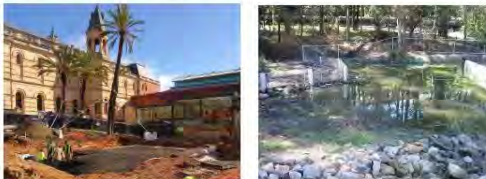
Figure 5: Stormwater storage being installed at the South Australian Museum (left), and stormwater harvesting pond at Barra Brui oval, St Ives (right).
