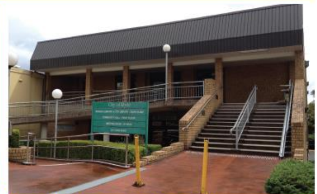
Existing North Ryde Library and School of Arts Community Centre
