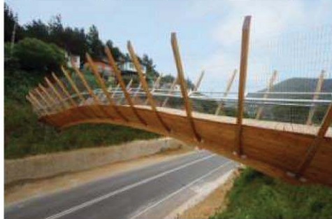
Figure 2 - Bridge by Tonkin Zulaikha Greer and Taylor Cullity Lethlean over Hume Highway, Melbourne
