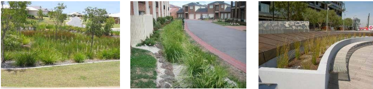
Figure 16 - Examples of bioretention systems in planter boxes, in the streetscape, and in parks
