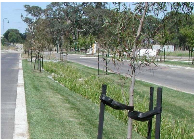
Figure 10: Typical swale and buffer strip configuration
