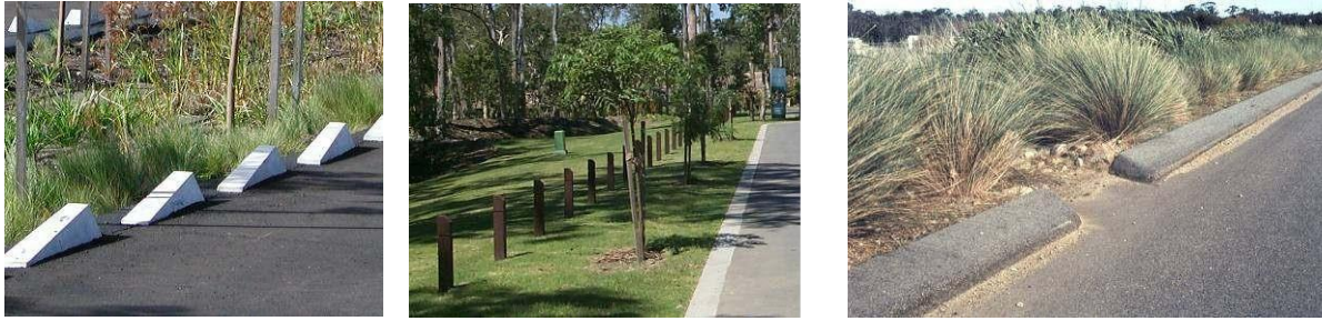
Figure 13: Different arrangements for delivering water to a swale and preventing vehicular access
