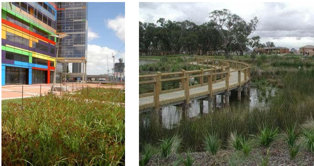
Figure 21 - Small and large-scale wetlands (Docklands and Lynbrook in Melbourne)
