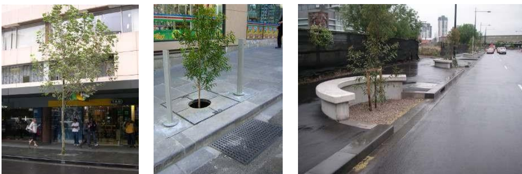
Figure 17 - Example street tree bioretention systems
