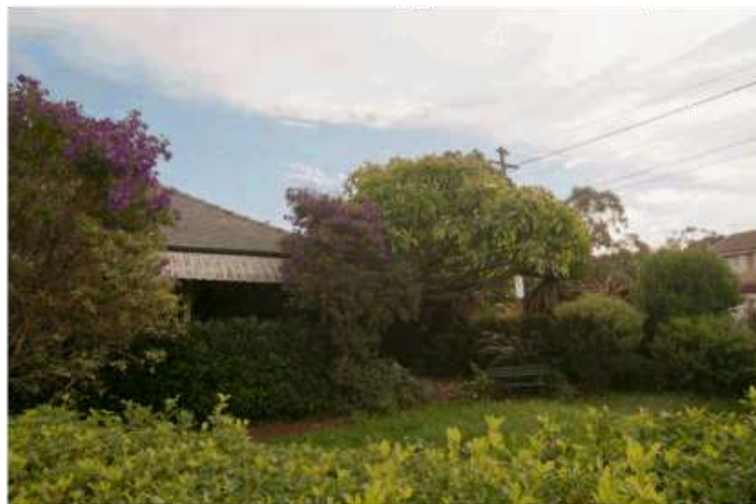
Figure 14: Detail of corner of the house with modern metal awning attached to front verandah and frangipani tree at the corner of the house.
