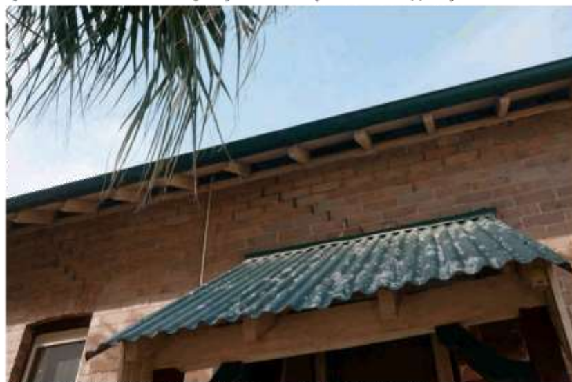
Figure 36: Settlement cracking at top of rear wall of the house arising from issues with damp proofing.
