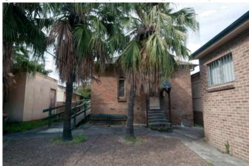
Figure 28: Detail of rear of house. Note evidence of rising damp to lower portion of rear wall
