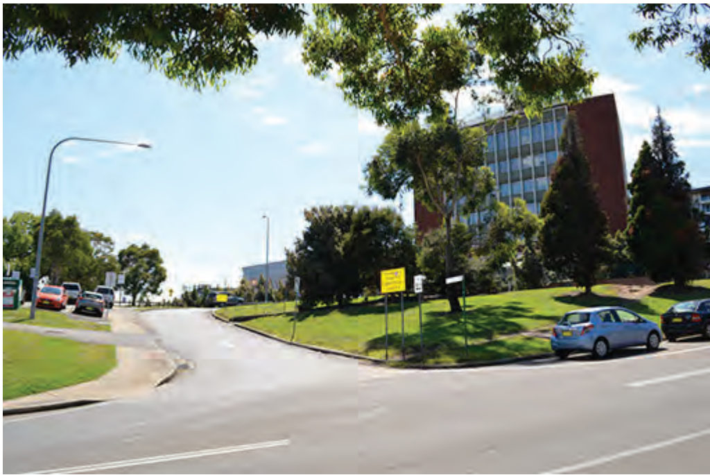
View from Parkes Street.JPG
