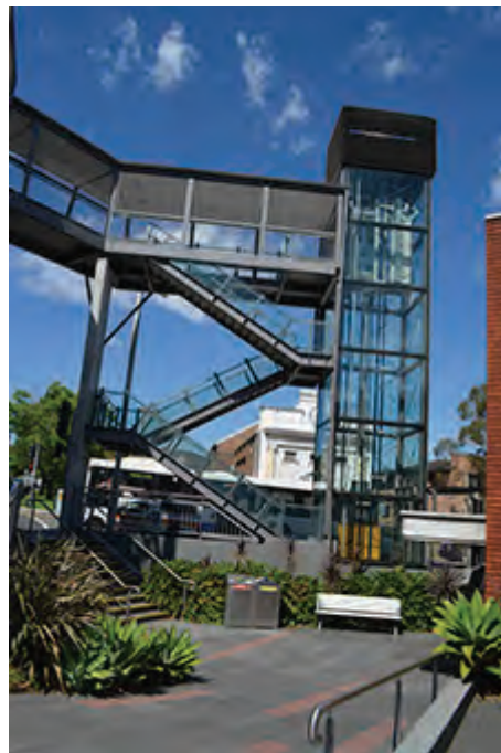
Southern Bridge Lift and Stairs.JPG
