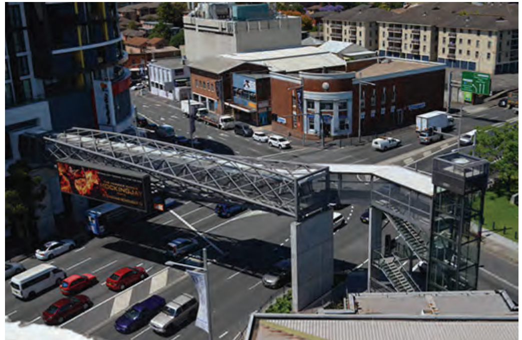
Southern Bridge setting.JPG
