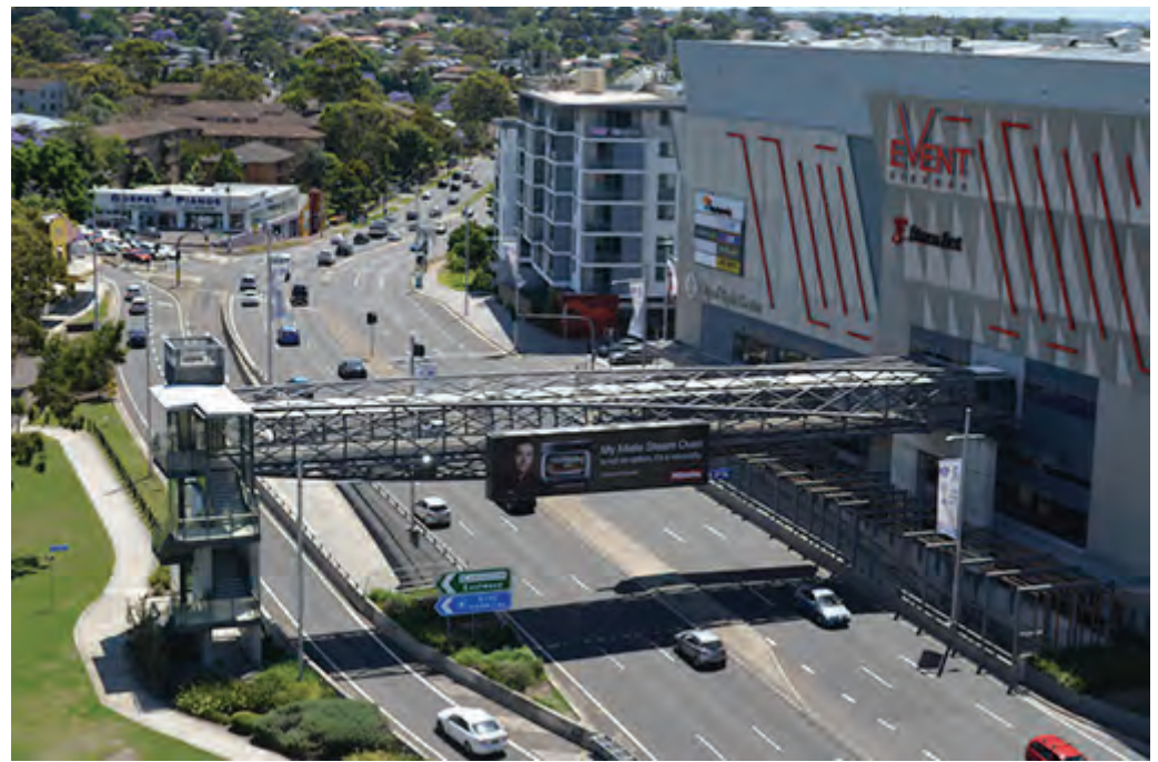
Northern Bridge setting.JPG
