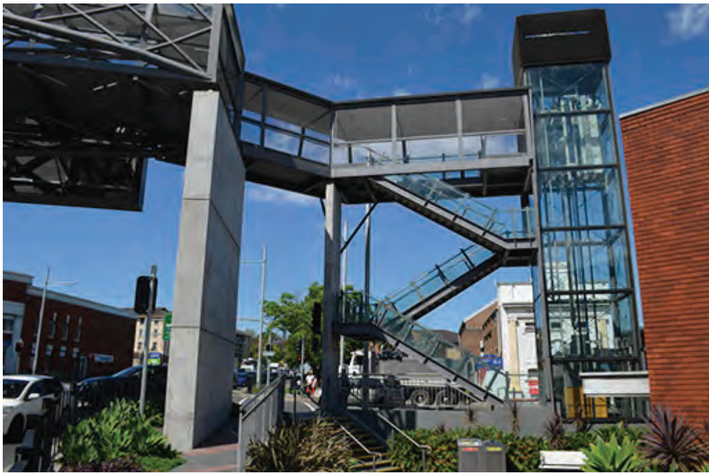
Southern Bridge West tower.JPG
