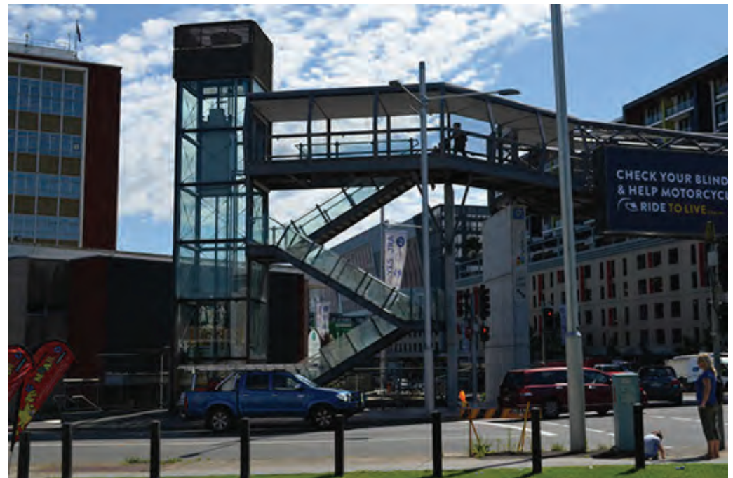
Southern Bridge West Tower from South.JPG
