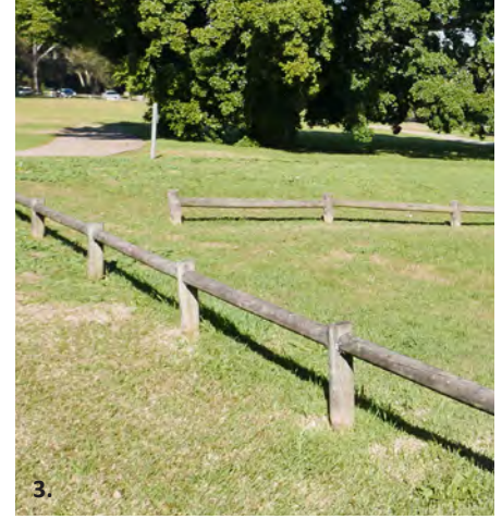
3. There is excessive boundary fencing between Bennelong Park and Kissing Point Park, and between the parks and the street.
