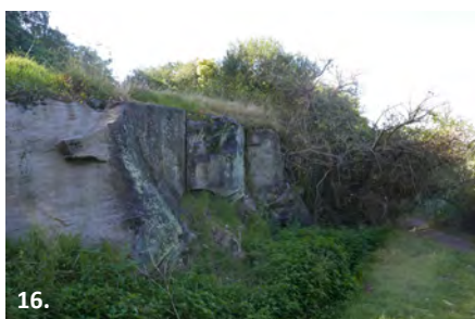
15. Punt Wharf remains are at Bedlam Point in Hunters Hill Council. They are a remnant of infrastructure associated with the Great North Road convict gangs and their crossing point at the Parramatta River.
