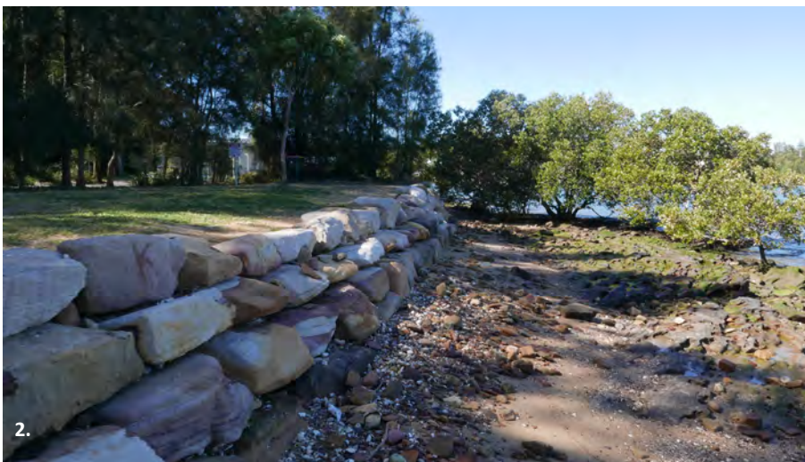
2. A small sandy beach at Memorial Park provides direct access to the river. The sea wall is constructed with sandstone blocks.
