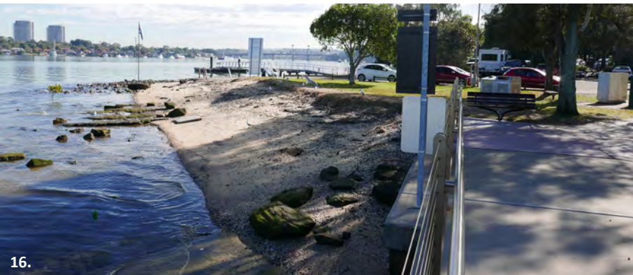
16. There is no foreshore pedestrian connection from the Rivercat wharf to the park.
