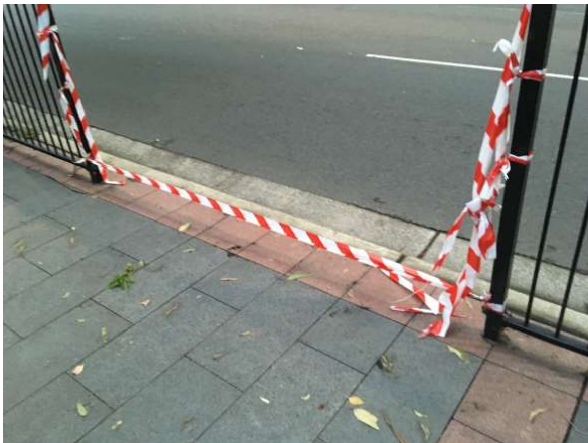
Above: Missing and damaged pedestrian fencing panels on Tucker Street
