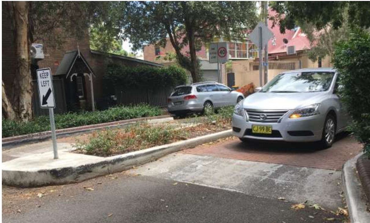
Photo 3: Raised threshold treatment
