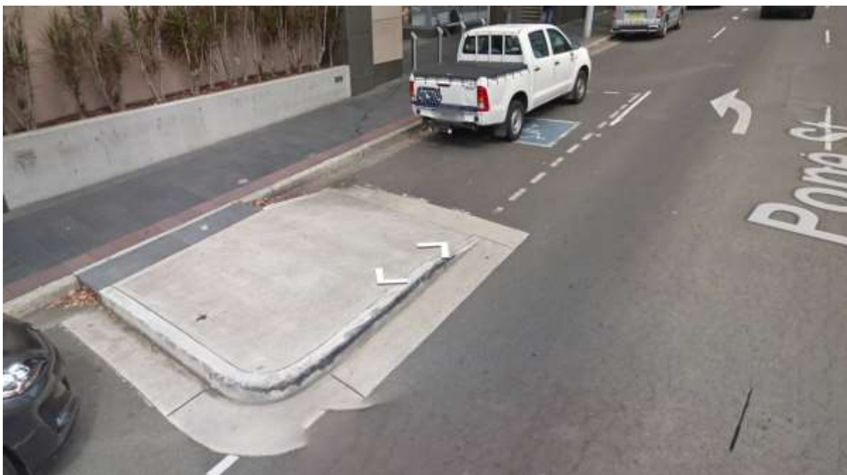
Photo 2: Existing kerbside traffic island associate with on-street accessible parking space, Pope Street.
