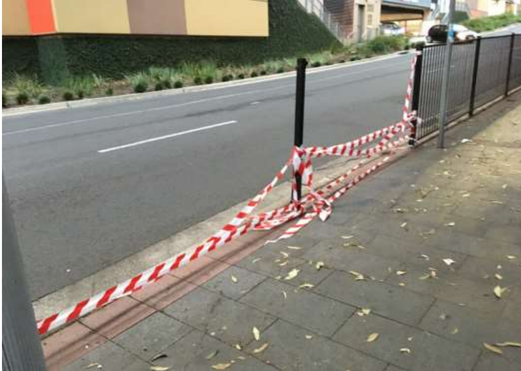
Below and above: Missing and damaged pedestrian fencing panels on Tucker Street
