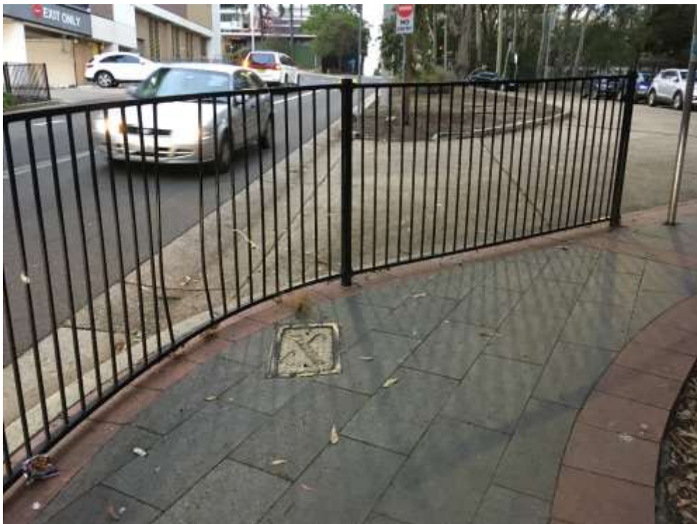
Below and above: Missing and damaged pedestrian fencing panels on Tucker Street
