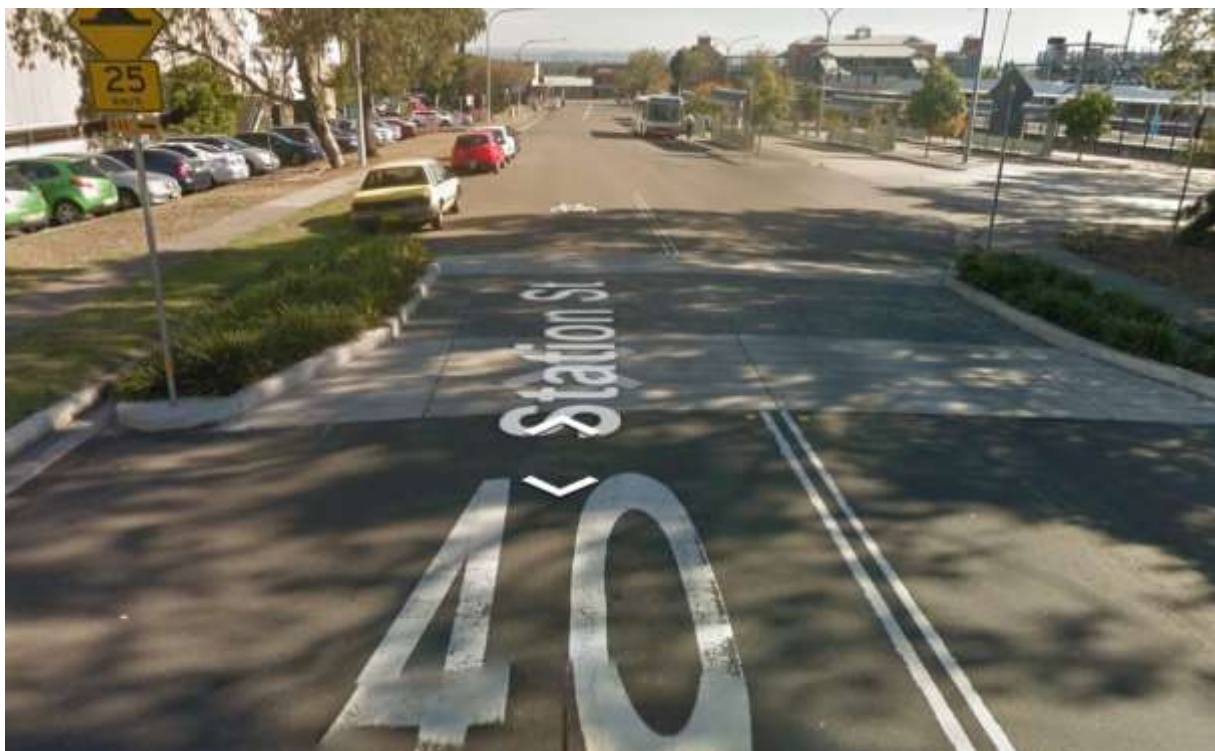
Photo 4: Raised threshold treatment
