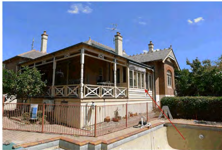
Figure 36: Kingsley taken from the south-east. The weatherboard kitchen extension onto the eastern verandah, is arrowed. The bay window with its gable end seen here at right is to the Formal dining room (see Figure below).
