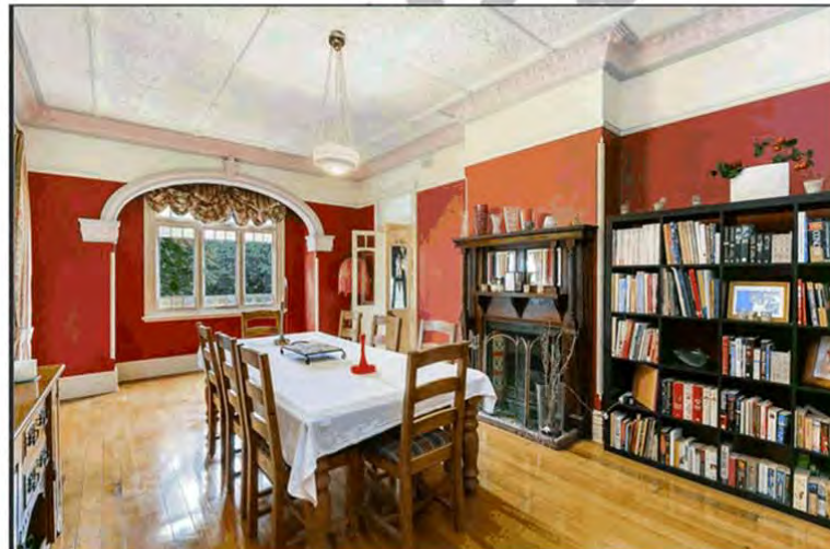
Figure 37: The formal dining room (centre of the east elevation of the house). Note the original decorative plaster panelled ceiling, decorative plaster cornices, picture rail, fireplace mantelpiece with Federation period tiles, timber flooring. The plaster arch draws attention to the bay window at the centre of the east elevation of the house. Image source:www.realestate.com
