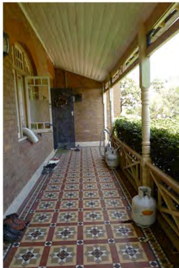
Figure 30: (Left) View along the northern verandah of Kingsley. Note tessellated tiling is recent (though sympathetic to the Federation period of the house). The decorative turned timber verandah posts and timber tongue and groove boarded verandah ceiling are original.
