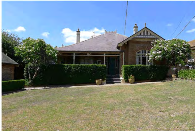
Figure 26: The north elevation of Kingsley facing Rowe Street (recent garage at left).
