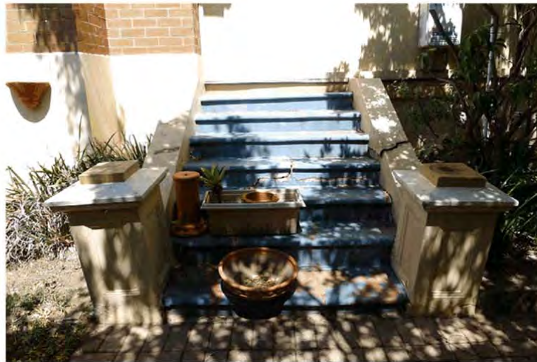
Figure 34: Original entry steps onto eastern verandah north of the central gabled bay. Some cracking is evident.
