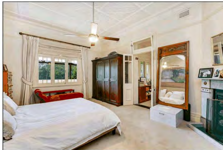
Figure 42: Interior of Bedroom 1 (north-east corner of the house), with original ceiling, cornices, picture rails, marble fireplace mantelpiece and original fireplace tiling. Note original timber panelled french doors and fanlight leading into the ensuite (the ensuite being a weatherboard partial enclosure of the east verandah). Image source:www.realestate.com
