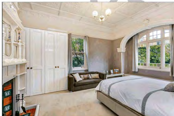
Figure 43: Interior of Bedroom 2 (north-west corner of the house), noting original ceiling, cornices, picture rail and (at left) timber fireplace mantelpiece with original fireplace tiling. The plaster arch draws attention to the bay window to the north elevation. Image source:www.realestate.com
